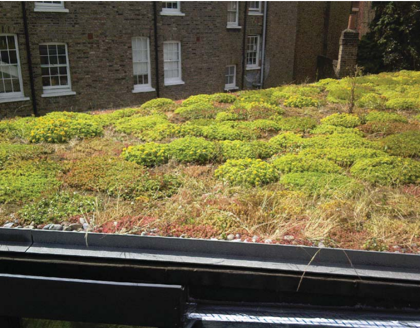
Typical extensive bio diverse green roof in residential environment
