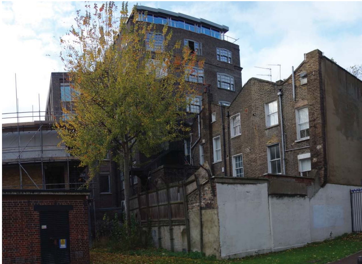
Rear elevation and garden walls with 10A Belmont Street in background
