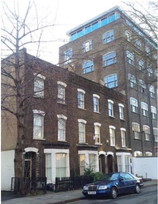
Current street view - 10-14 Belmont Street
