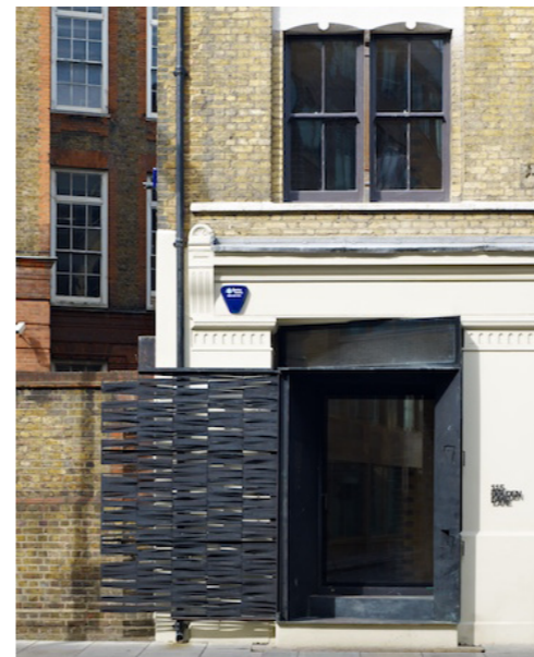
Fig. 35 - Period warehouse refurbishment. Folded & perforate brass screen, patinated dark brown (A). Brick cleaned of all paint and lightly sootwashed (B). Original timber windows reinstated and painted (C).
