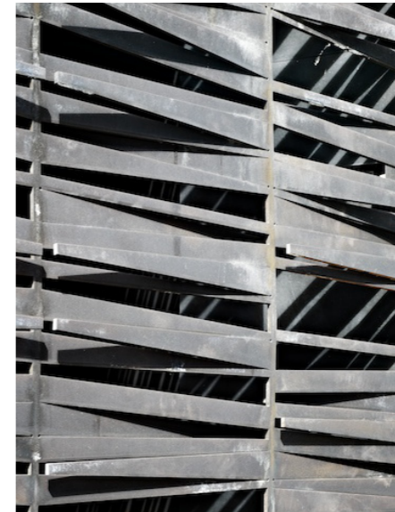
Fig. 33 - Folded & perforate brass screen, patinated dark brown (A)
