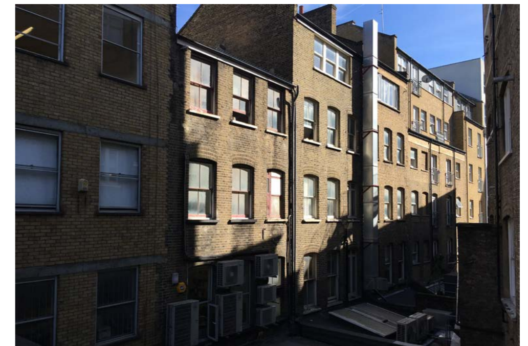
Fig. 12 - Rear elevation of 47-37 Farringdon Road
