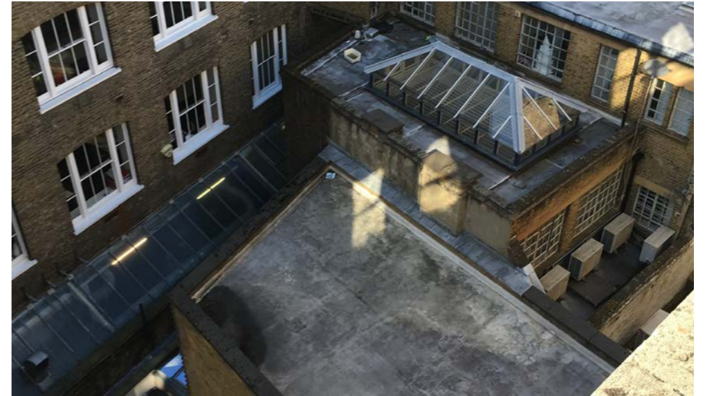
Fig. 16 - Rear roofscape of 51 Farringdon Road & 1 Lily Place
