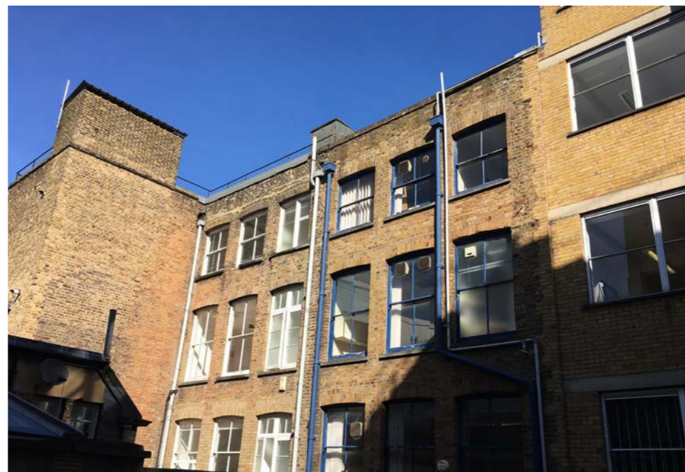
Fig. 11 - Rear elevation of 53 & 57 Farringdon Road
