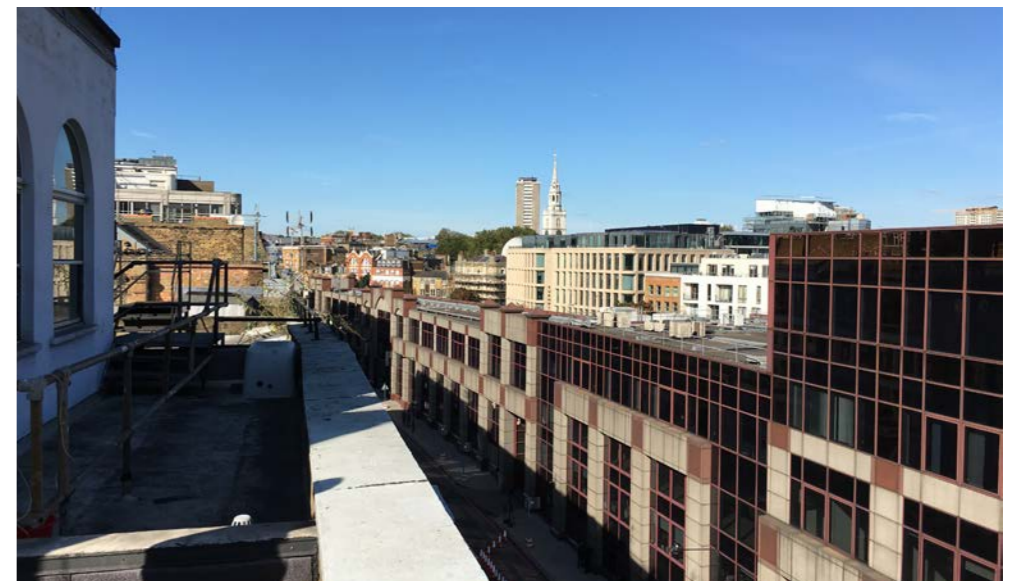
Fig. 18 - Farringdon Road roofscape, looking north from site
