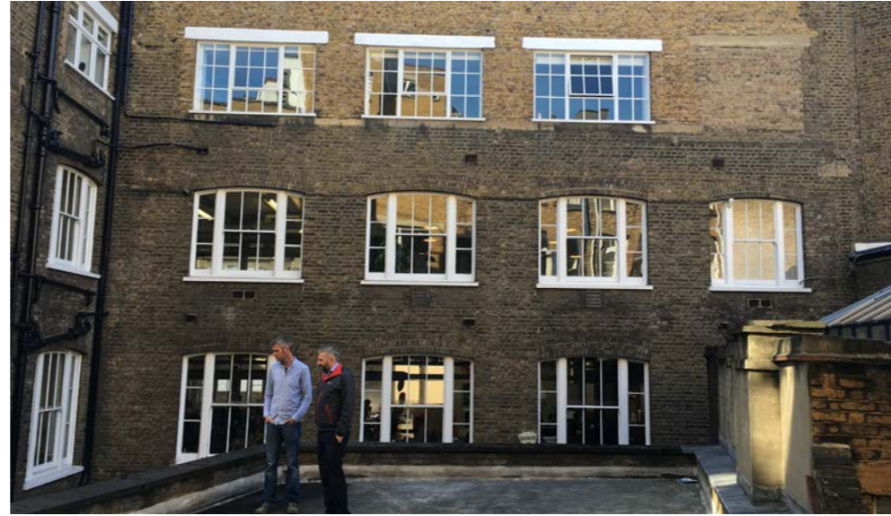
Fig. 13 - Rear elevation of 32-38 Saffron Hill, from 1st floor
