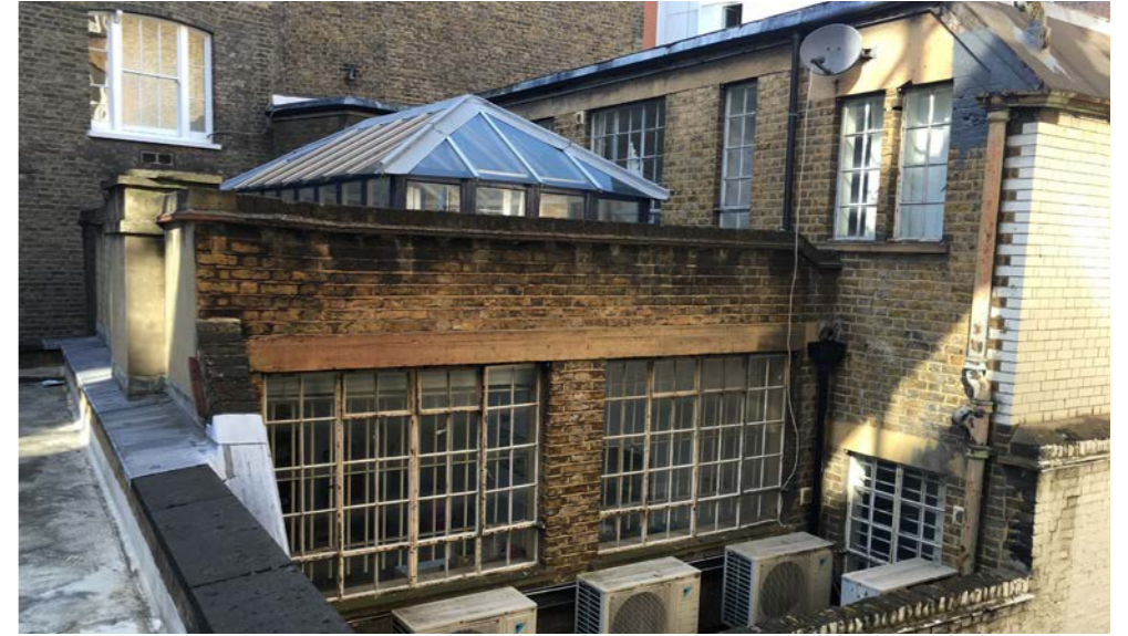
Fig. 14 - Rear elevation of 1 Lily Place, from 1st floor roof.
