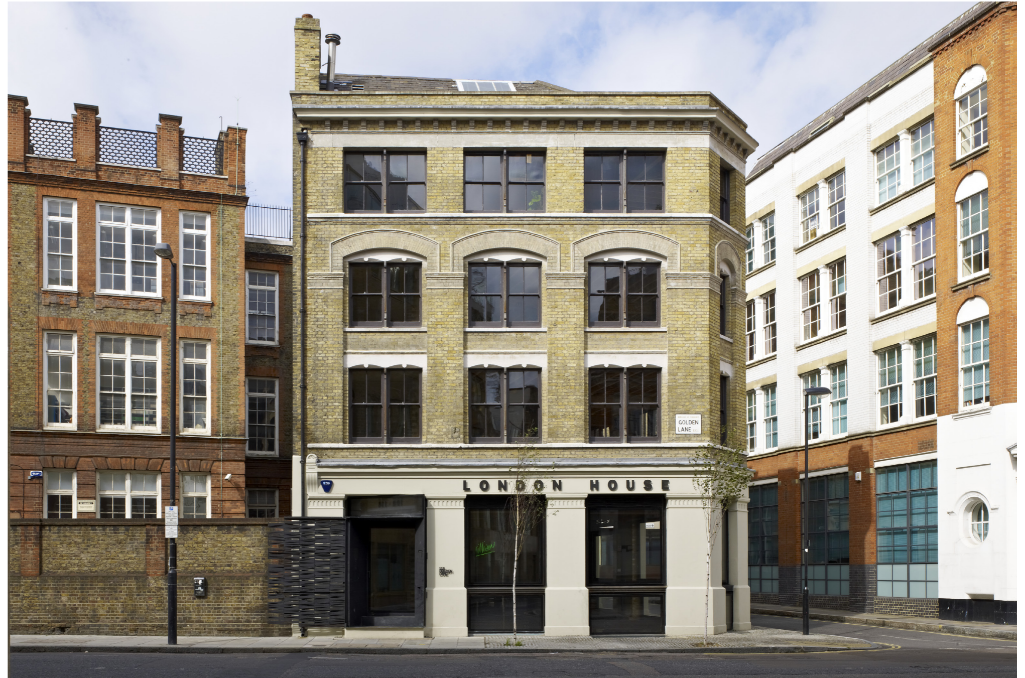
Golden Lane facade
