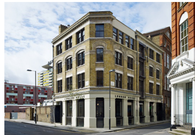
Golden Lane facade
