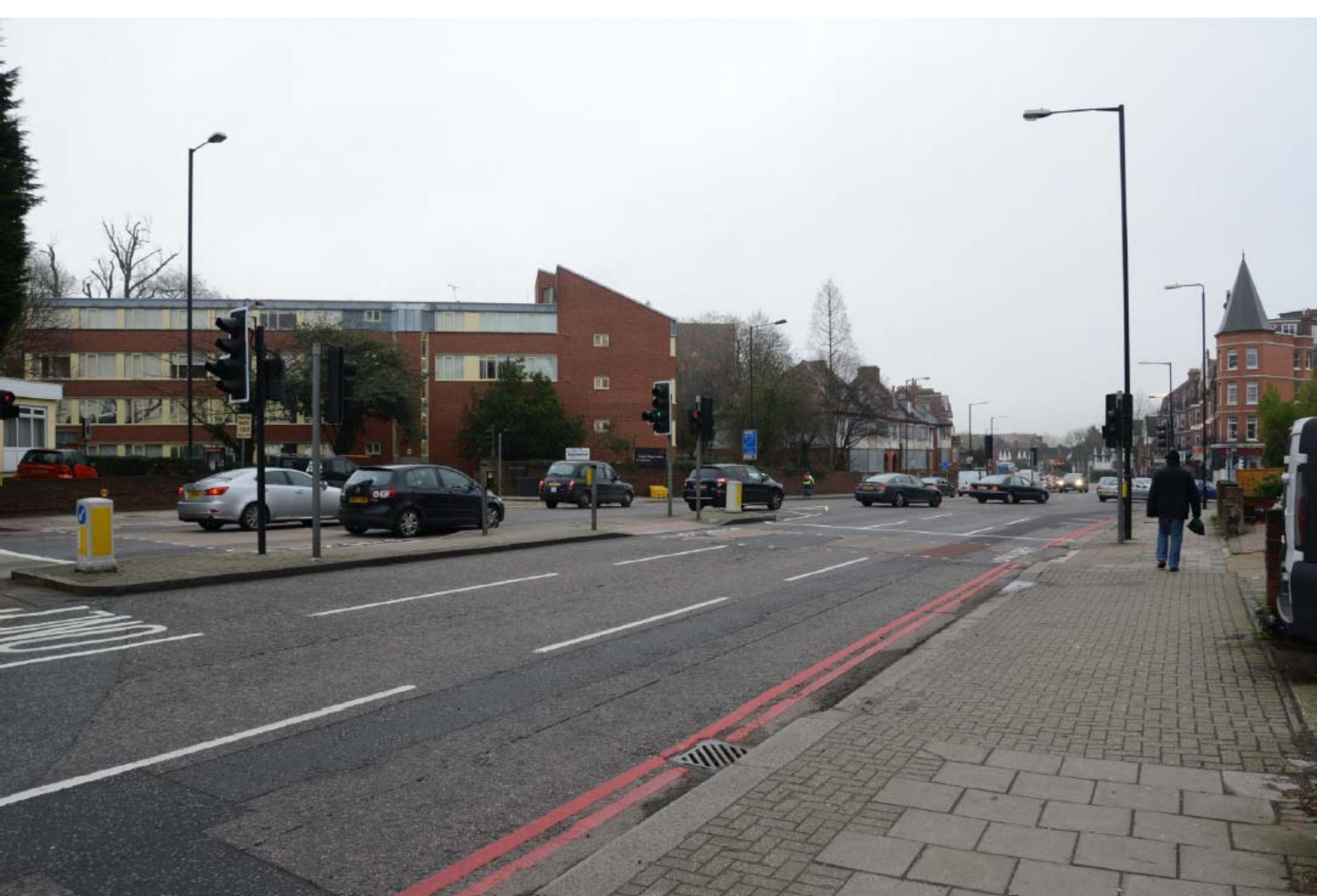
Existing view from Finchley Road looking to Platt's Lane junction
