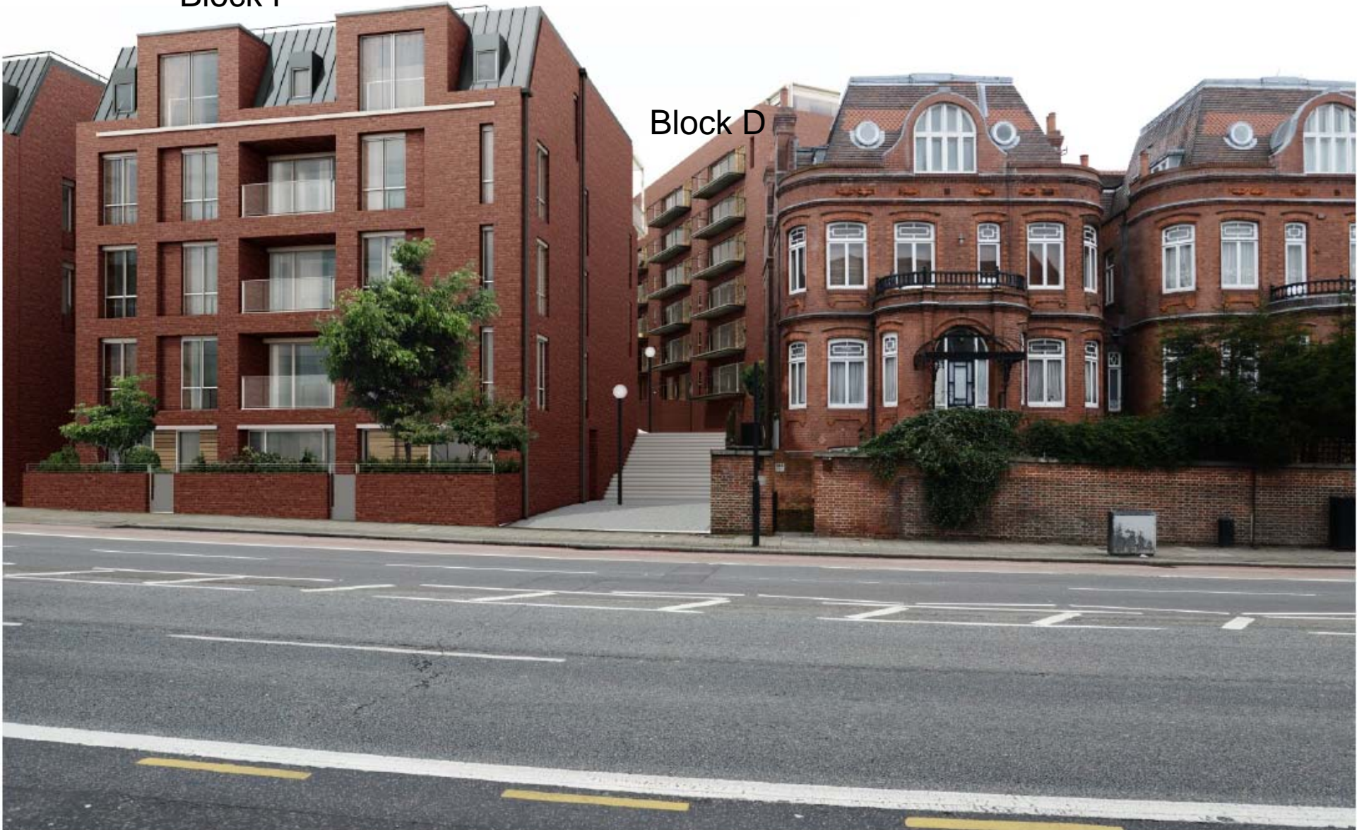
Proposed view from Finchley Rd: new block F and refurbished library becoming block D
