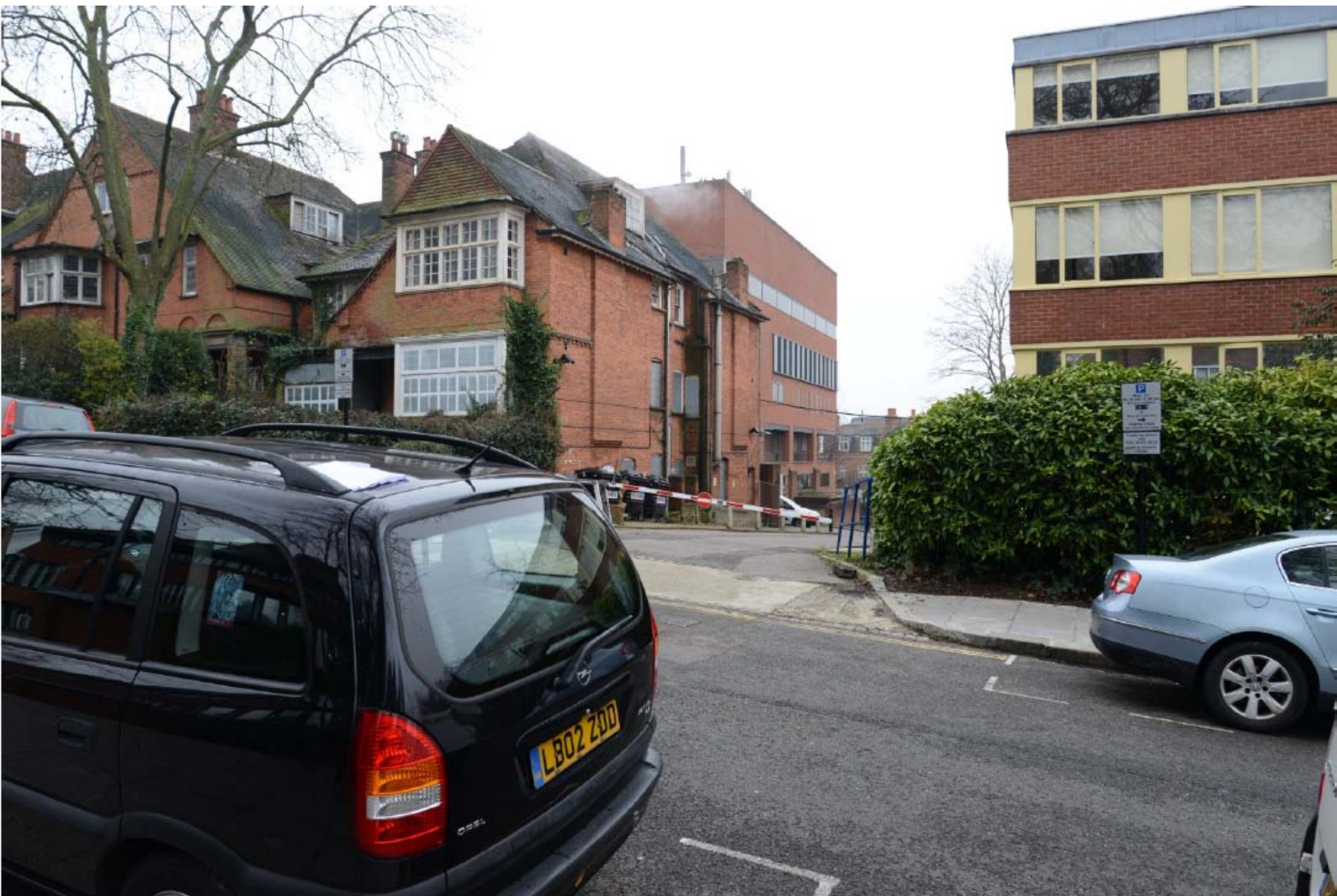
Existing view from Kidderpore Avenue, looking towards library (block D)
