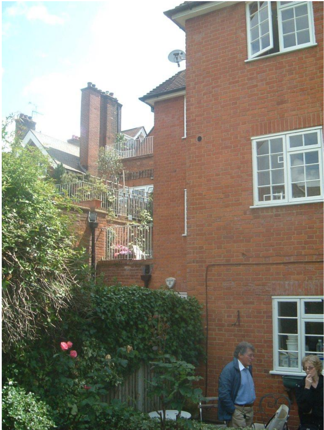
Figure 4 – View of neighboring property at No. 26 Eton Avenue
