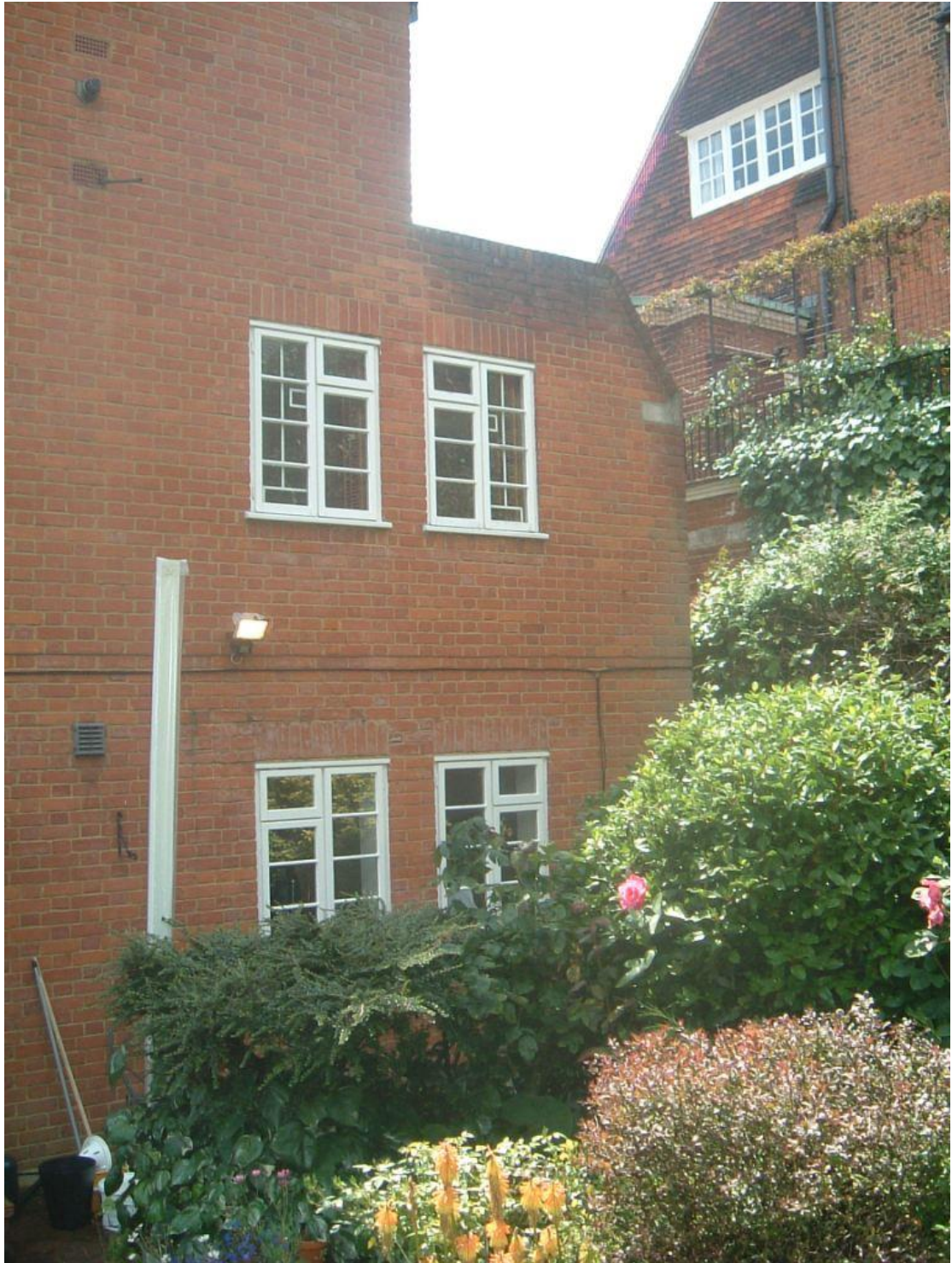
Figure 1 – View of existing extension to the rear.
