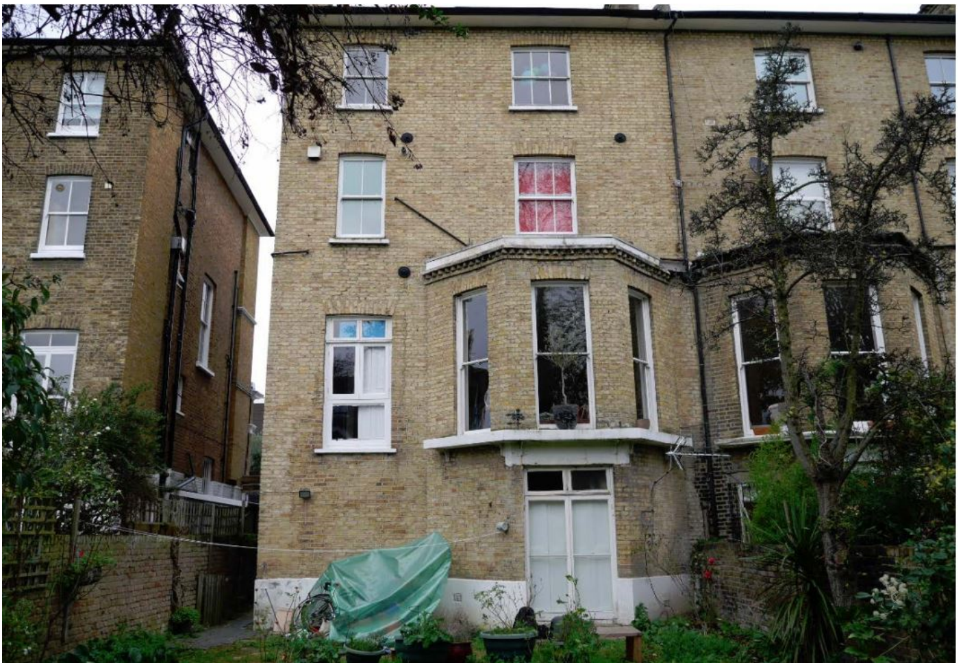
3. View to the rear of the property
