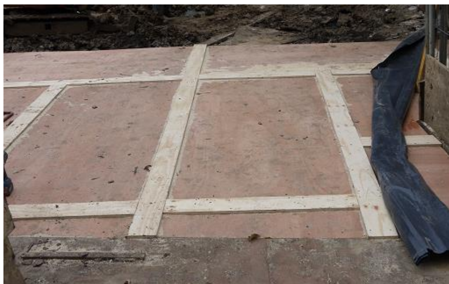
Figure 7. Plywood sheeting used as ground protection.
