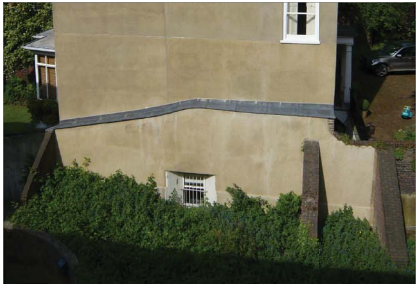
5 Photo of existing buttress and windows
