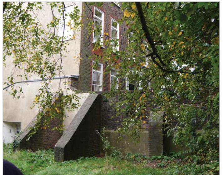
4 Photo of existing buttress
