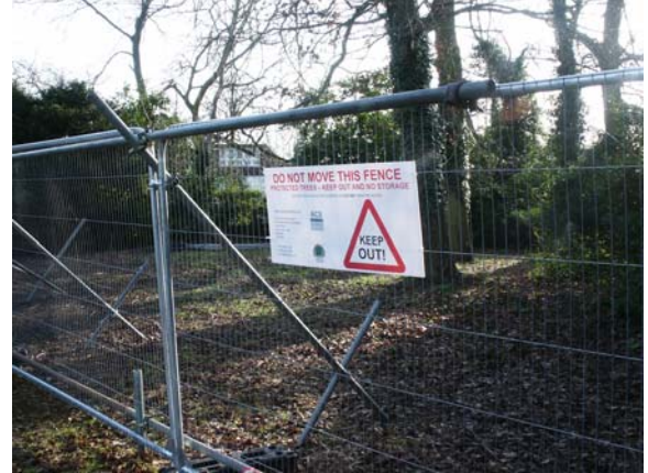
Effective fencing in position
