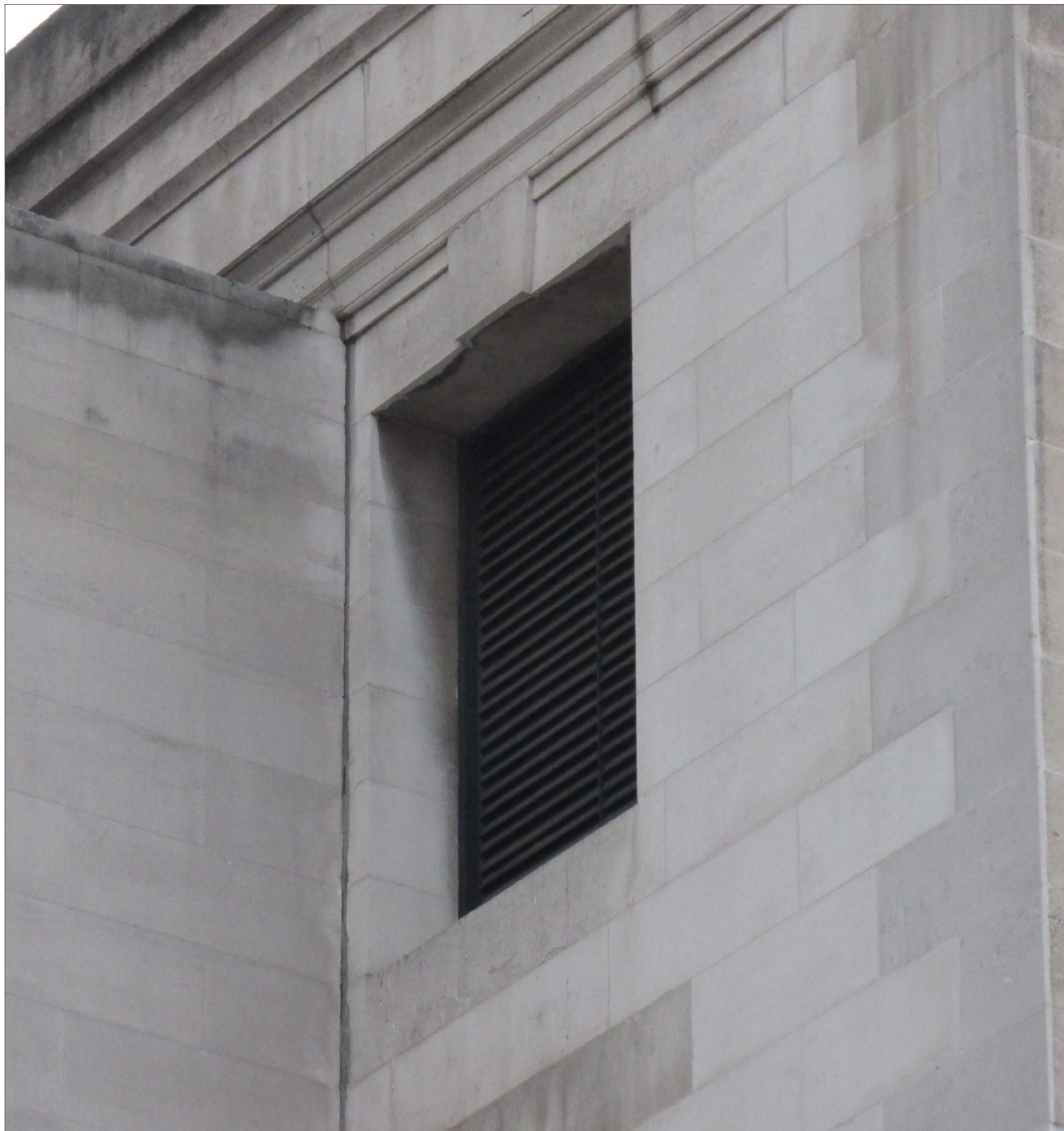
A Existing Window with louvre system Site Photo
