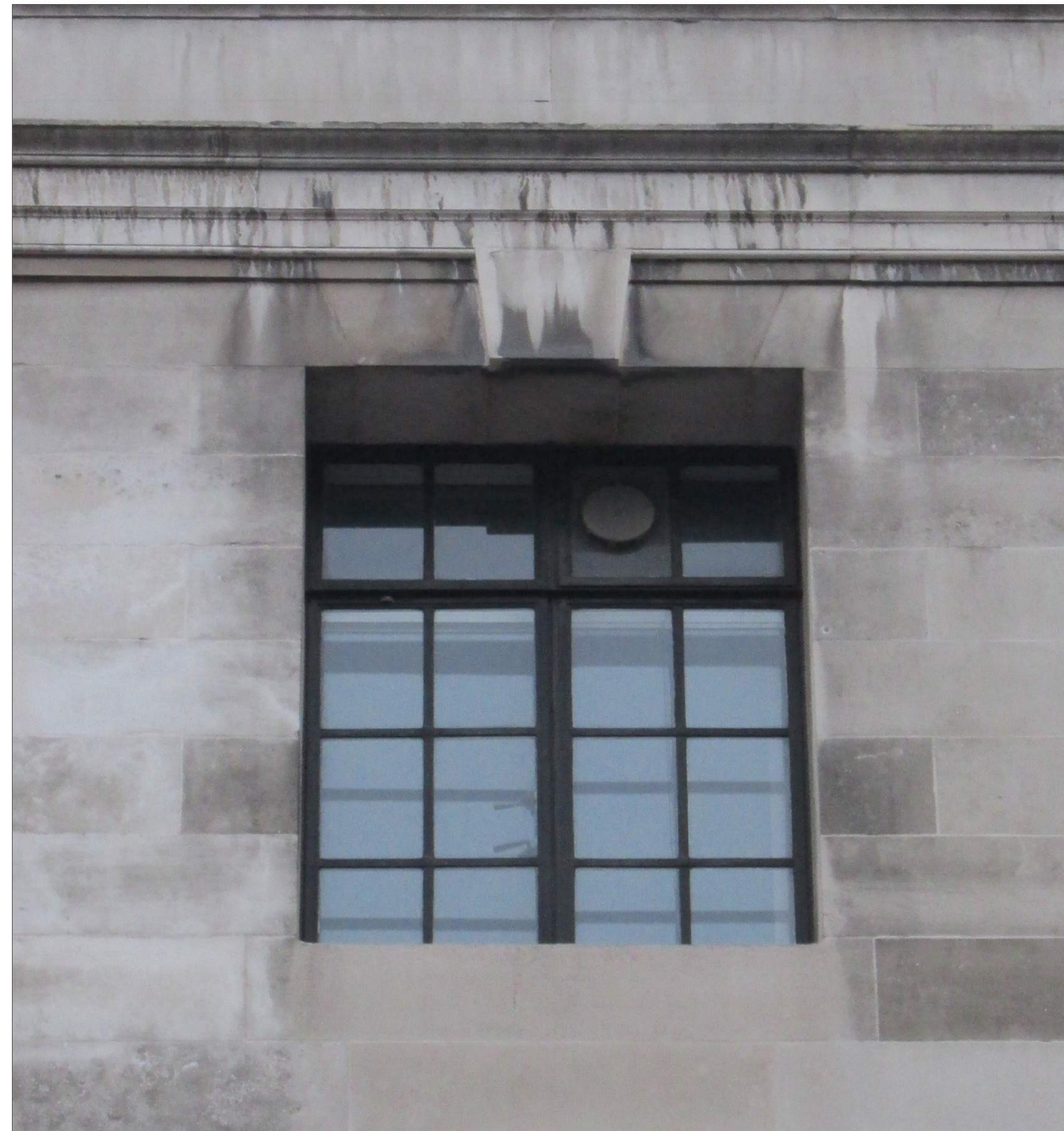
B Existing Third Floor Metal Frame Window Site Photo
