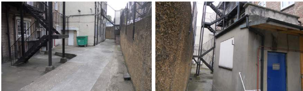
Existing site conditions
