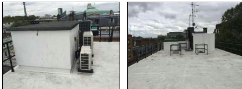
Photographs 1 and 2 – Existing Roof
