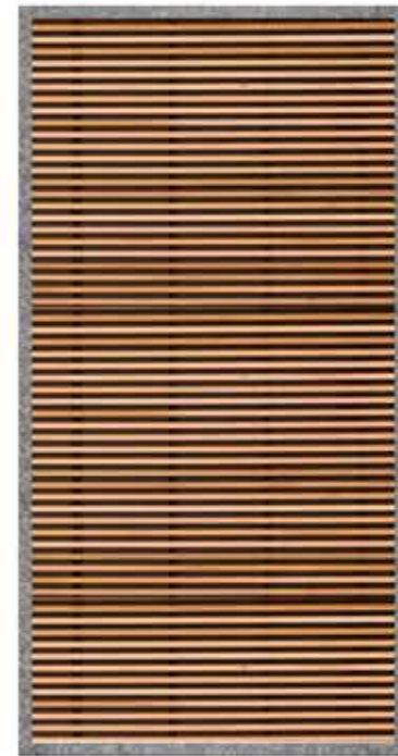
Galvanised steel frame and horizontal timber slats
