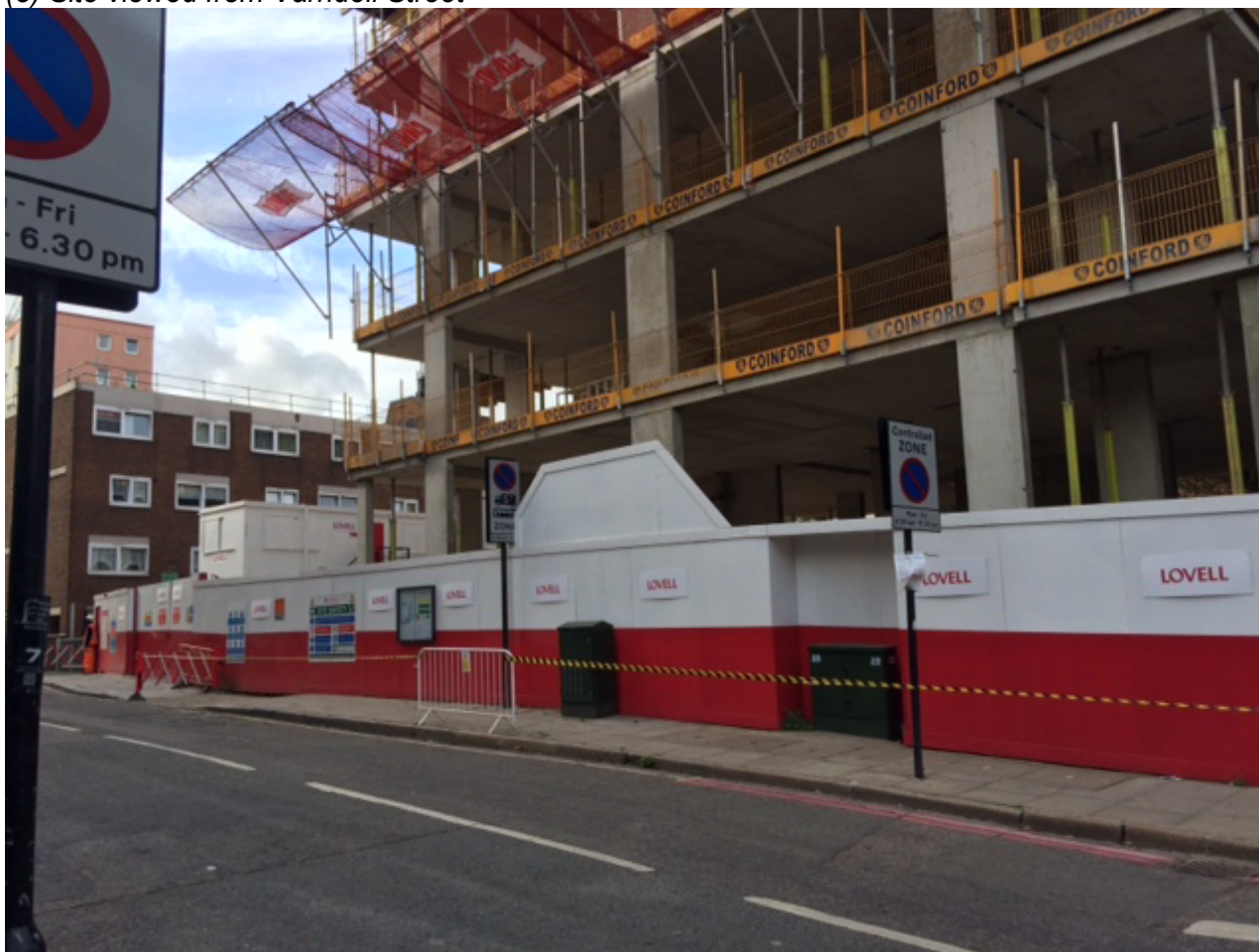
(5) Site viewed from Varndell Street
