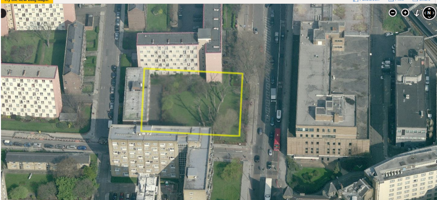
(1) Aerial photo #1 (Prior to commencement of works)
