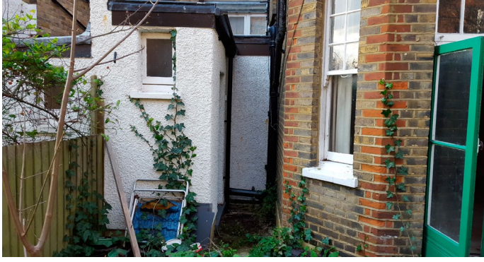
Above: Existing infill extension
