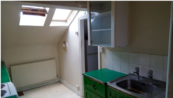
Above: Second floor kitchenette- location of proposed dormer
