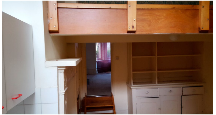
Above: Redundant ground floor kitchen mezzanine
