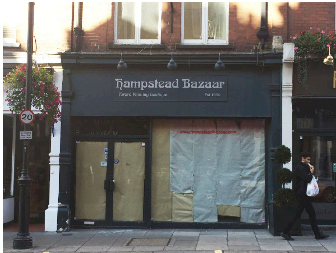
Photo of Existing Shopfront Elevation
