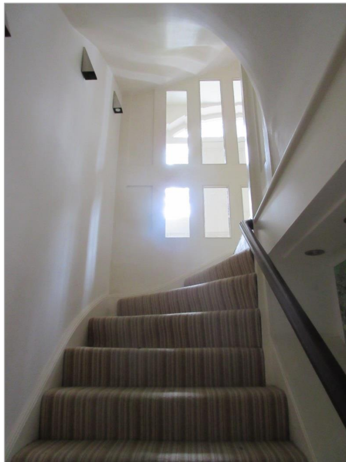
4h: Stair from lower ground to ground floor
