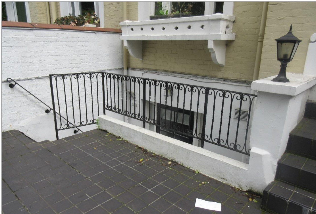
4a: Front garden, showing modern tiling, light fittings and railings to light well/area
