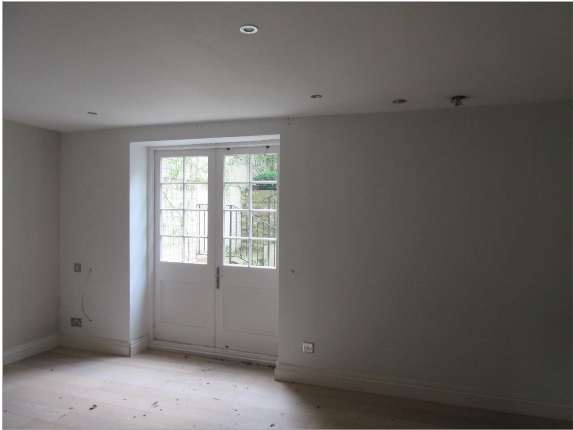
4g: Lower ground floor view towards garden
