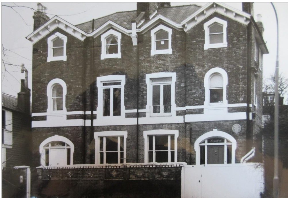
Figure 3: Exterior in 1970 (GLC/English Heritage)
