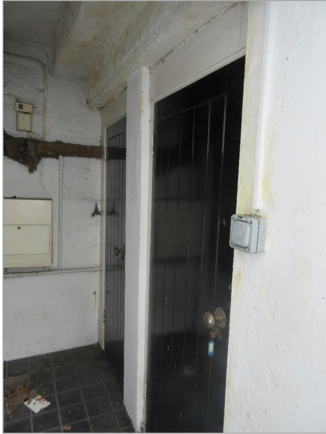
4c: Doors to vaults under entrance steps
