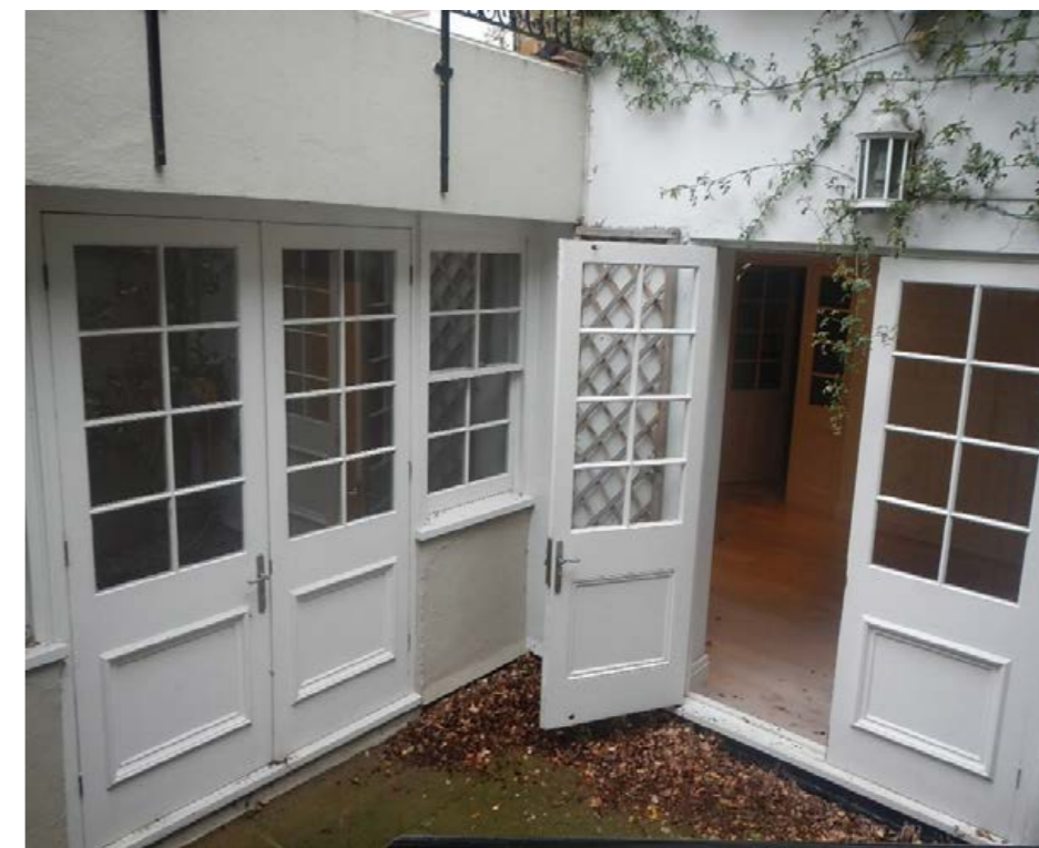
Fig.13: 17 East Heath Road - Rear Lower Ground
