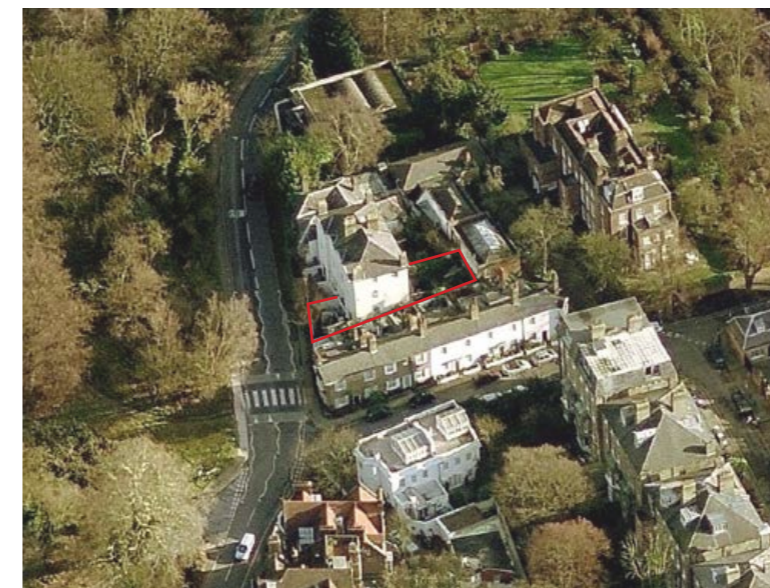
East Heath Road & Surroundings Aerial View 02 (Site outlined in red)
