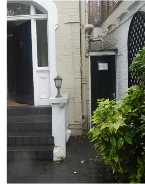
Fig.03: 17 East Heath Road - Storage Shed to Side Passage
