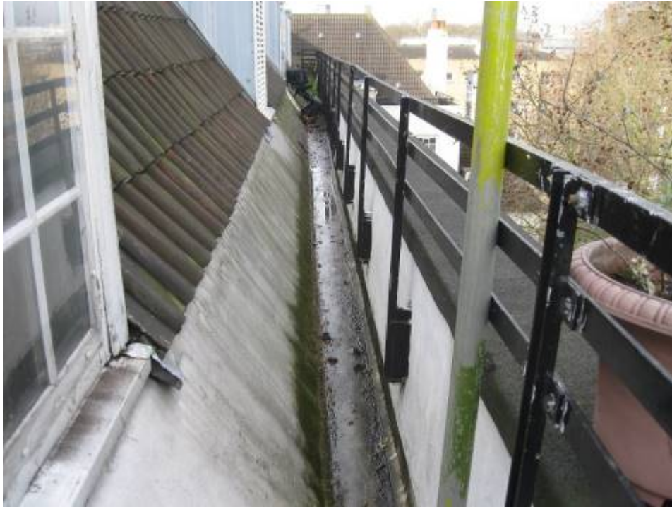
Photograph 17 Parapet Gutter
