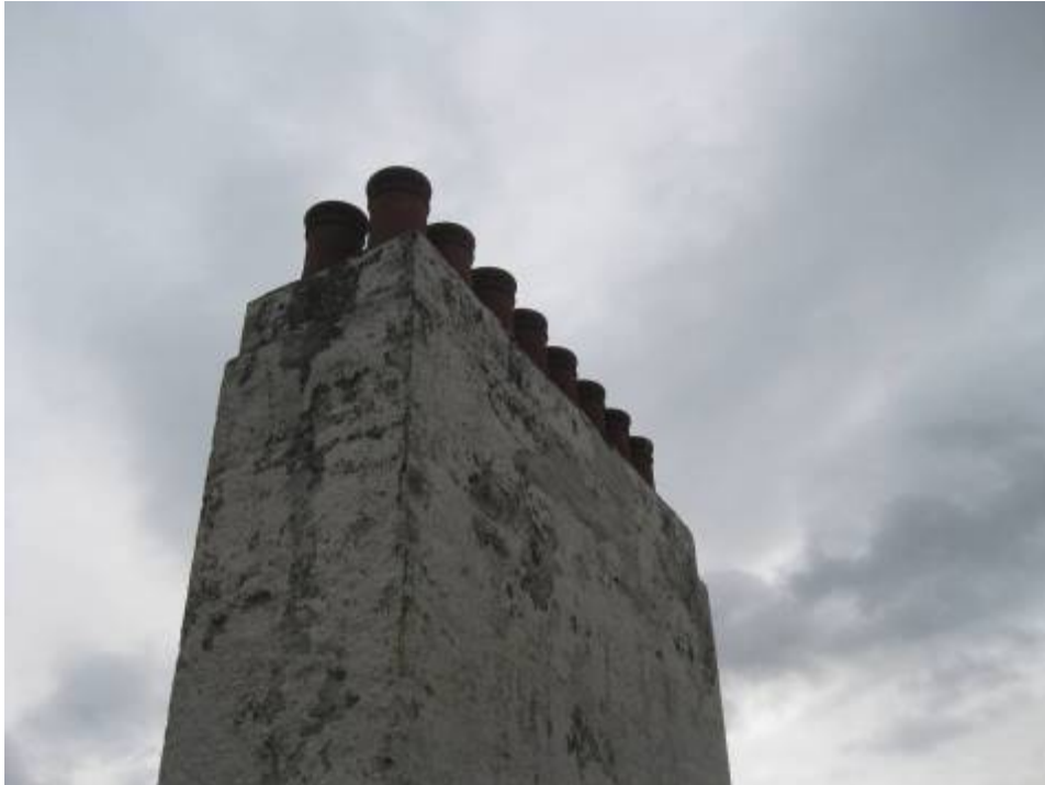
Photograph 21 Typical chimney condition
