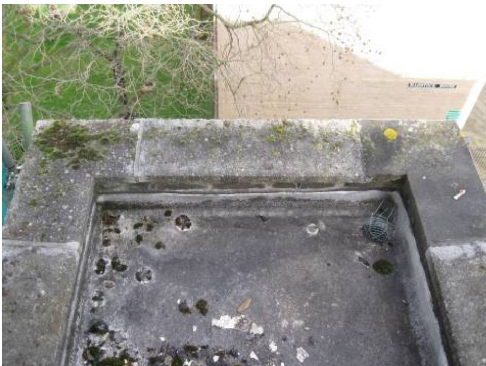
Photograph 20 Small flat roof area 204 - 238
