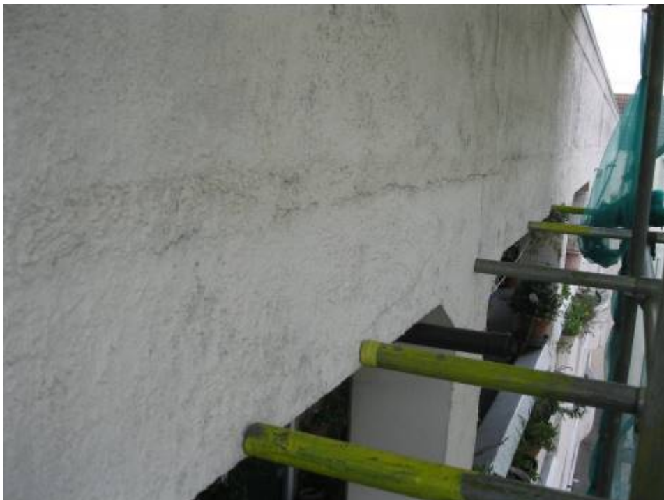
Photograph 22 Cracking to access balcony ring beam and render
