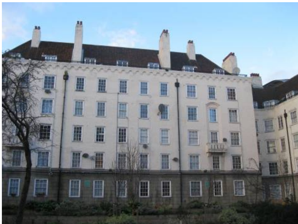
Photograph 4 Rear 204 – 238, courtyard side.
