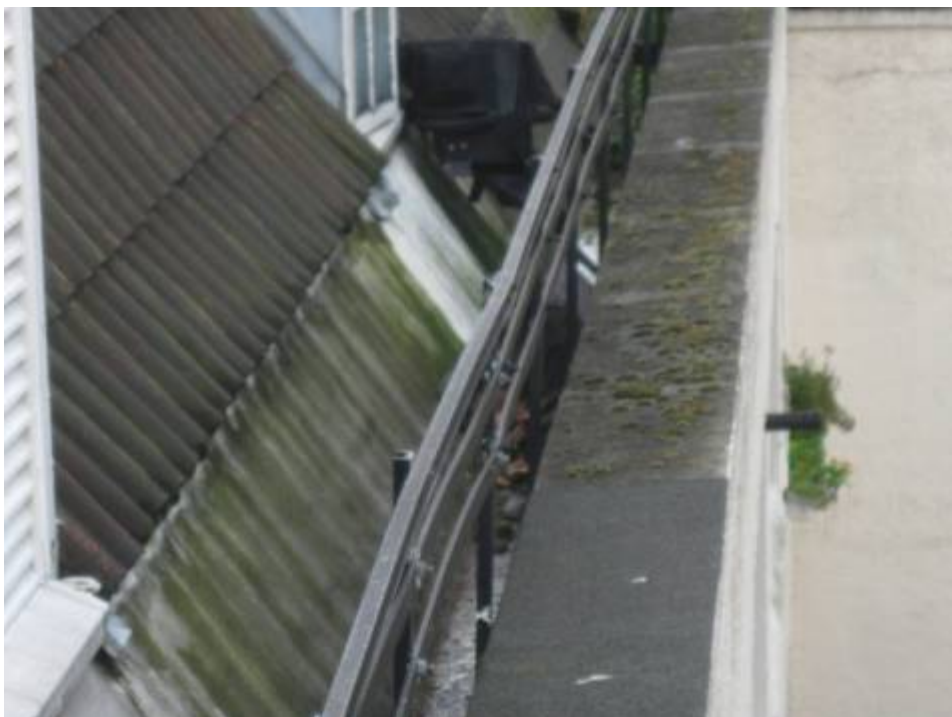
Photograph 16 Parapet gutter and coping
