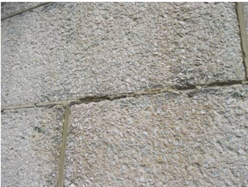
Photograph 34 Defective pointing
