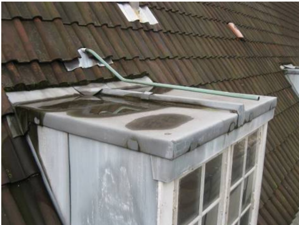
Photograph 18 Zinc clad dormer
