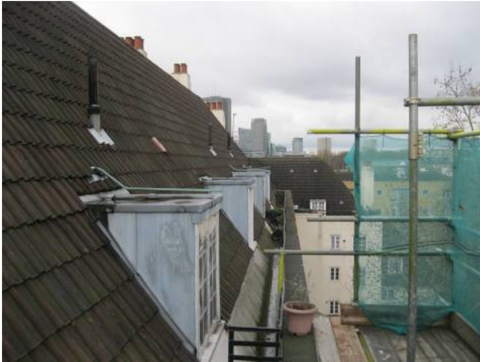
Photograph 15 Parapet gutter and dormers 204 - 238
