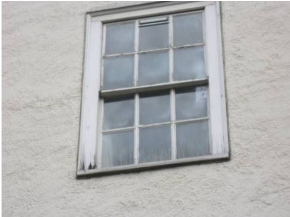
Photograph 29 Window condition, note low level decay
