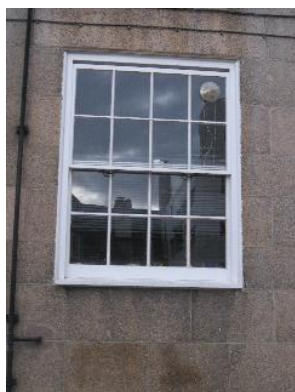
Existing sash window
