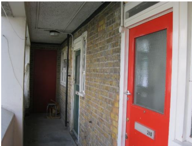
Existing Levita entrance door.
