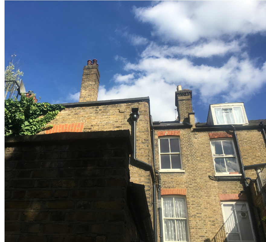
Rear view showing back elevation
