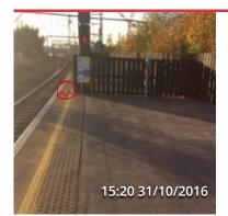
ISSUE 1 WILLESDEN END OF PLATFORM NO2 Existing fence to remain unchanged Install Rosehill anti trespass panel only between fence and end of platform
