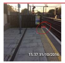
ISSUE 3 WILLESDEN END OF PLATFORM NO1 Existing fence to remain unchanged Exchange existing precast concrete anti trespass panel for Rosehill type anti trespass panel
