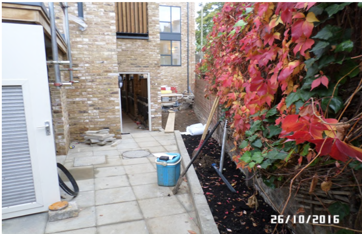
Photograph 1 – View north along the eastern boundary towards TP1.
