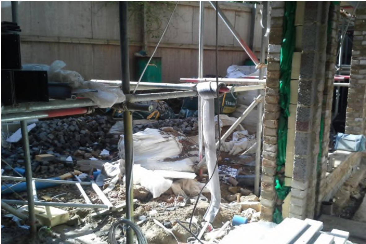
Photograph C– View north towards the northern boundary.
