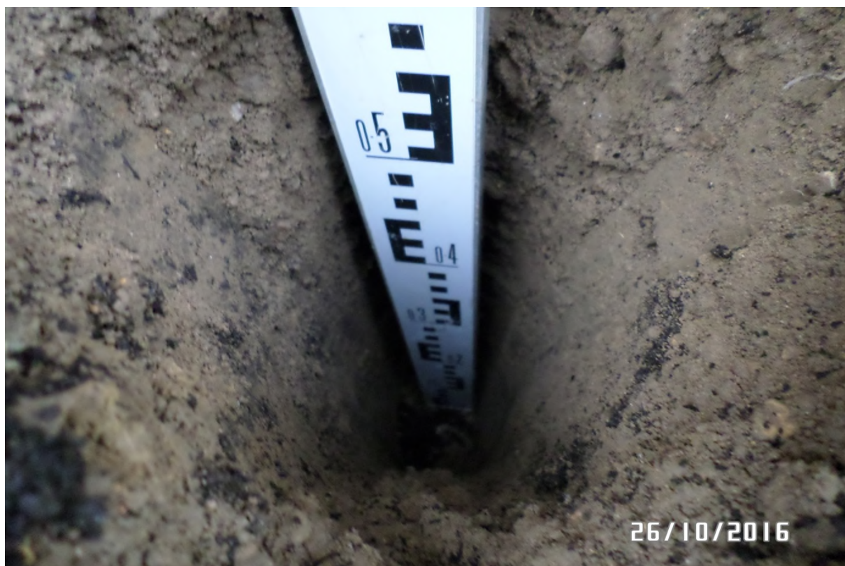
Photograph 4 – View of TP2.
