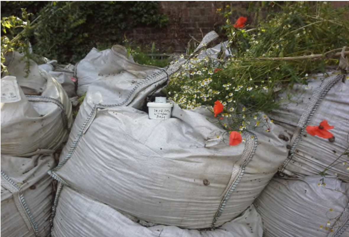
Photograph D – View of stockpiled imported Topsoil.
