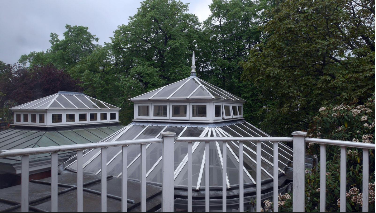
Conservatory roof (centre) at rear of house
