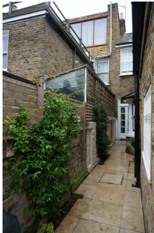
Existing side passageway
