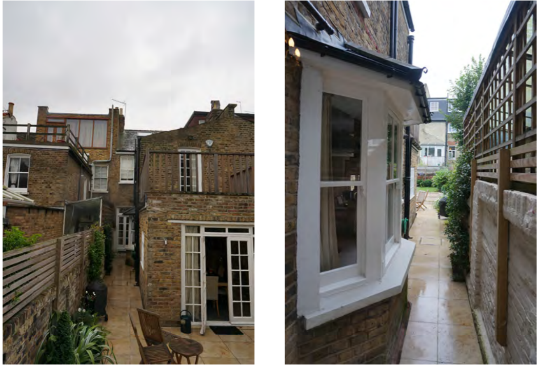
Views of existing side passway and back extension at 66 Solent Rd, dormer extension at neighbouring property 64 Solent Rd
