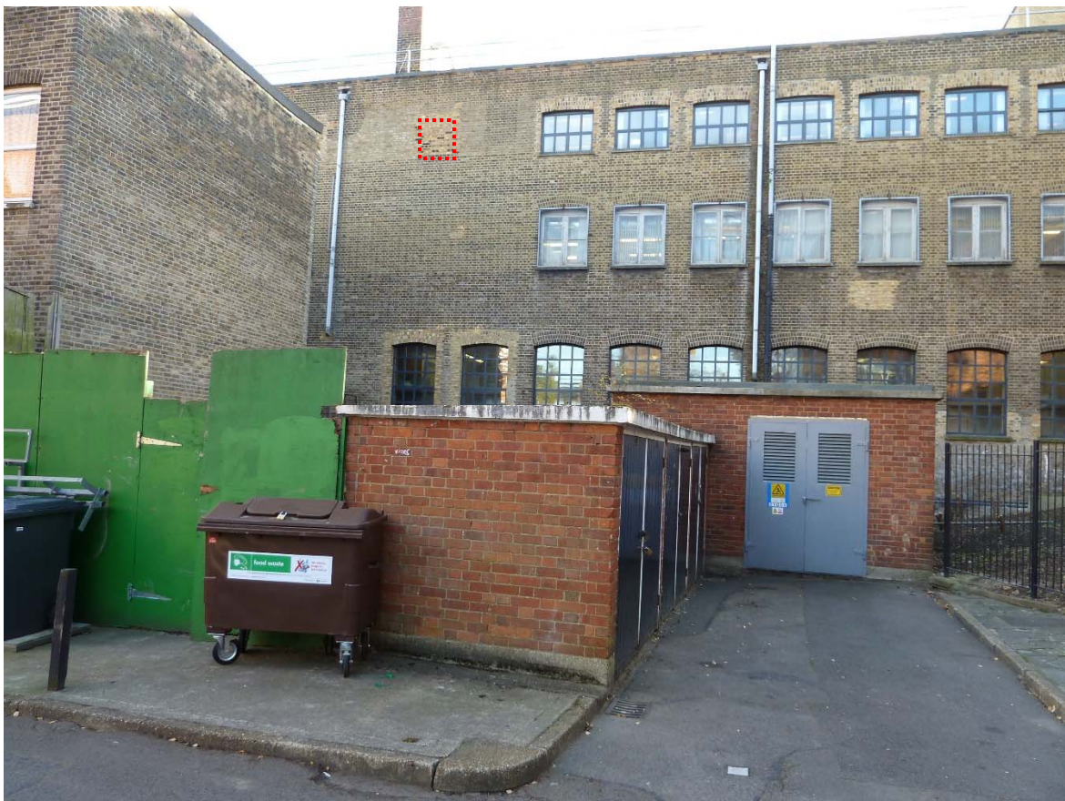
Photo 1 – North Elevation (from Kilburn Vale Estate).
