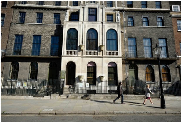
Figure 4: Existing signage to railings, May 2016
