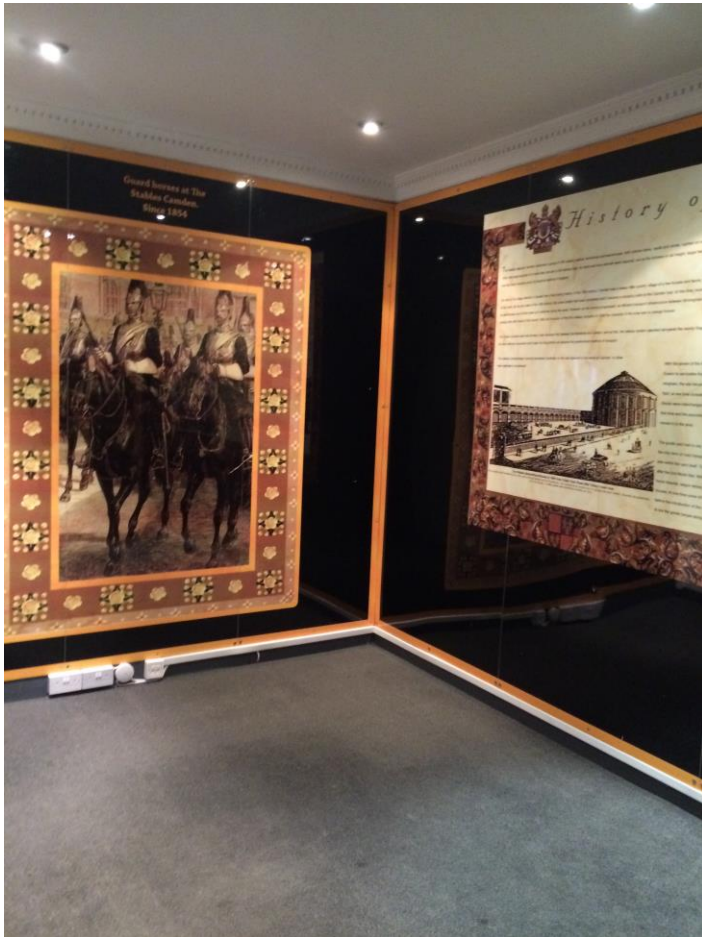
Figure 7: Tack Room: first floor: north bay. Modern wall linings, partitions and suspended plasterboard ceiling to be removed.
