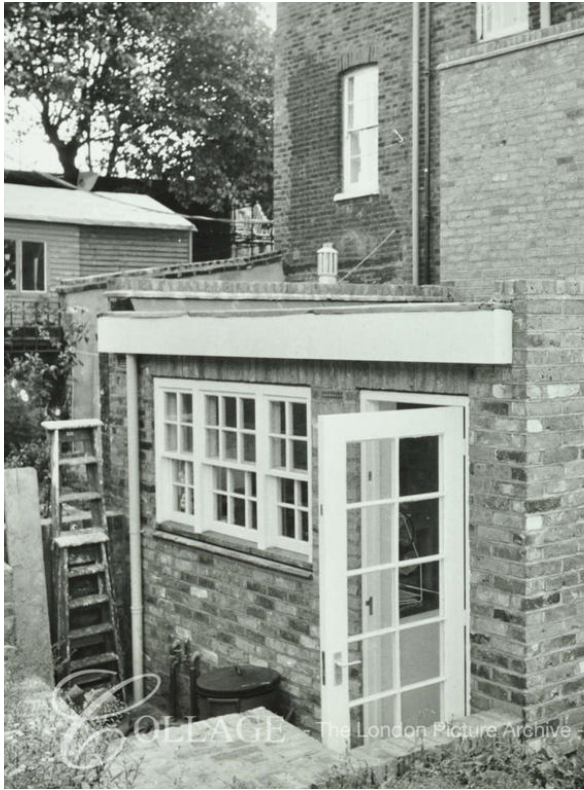
Figure 14/ Rear of No.s 7-8 Little Green Street, 1970 © London Metropolitan Archive.
