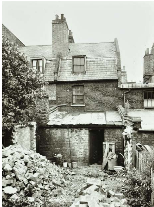
Figure 11/ Rear of No.s 7-5 Little Green Street, 1968 © London Metropolitan Archive.
