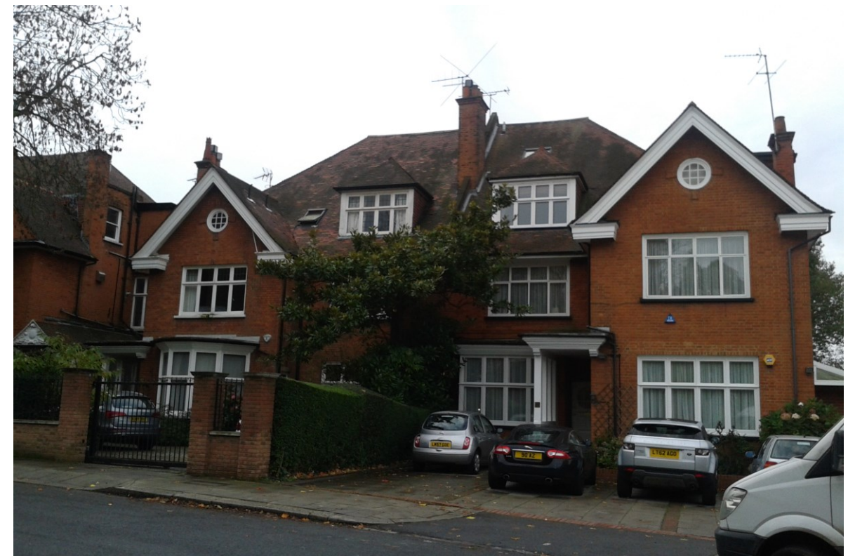
Figure 25 A photograph of typical semidetached dwellings within the Redington and Frognal Conservation Area.
