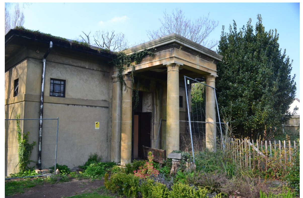
Figure 109. A photograph of the Chapel from the southeast, showing the Doric portico to the east elevation.
