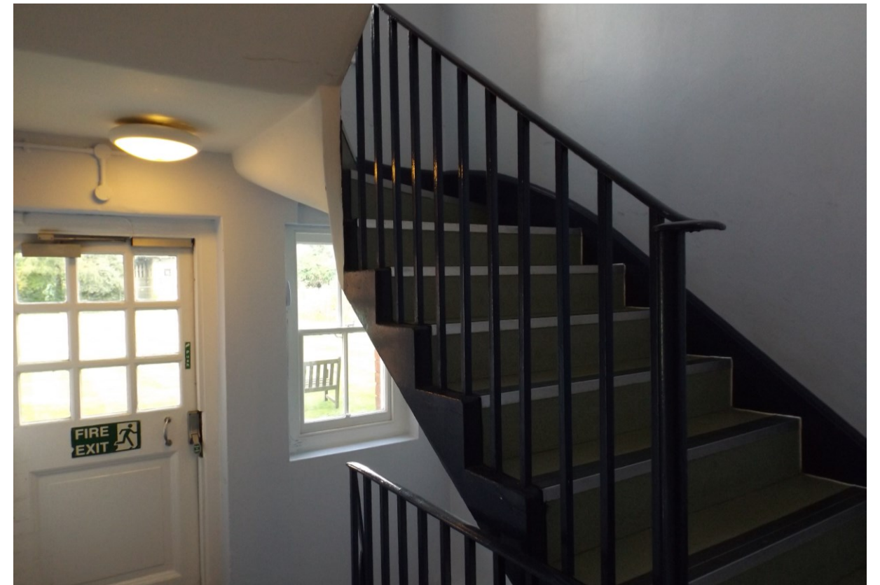
Figure 85. The internal staircase.
