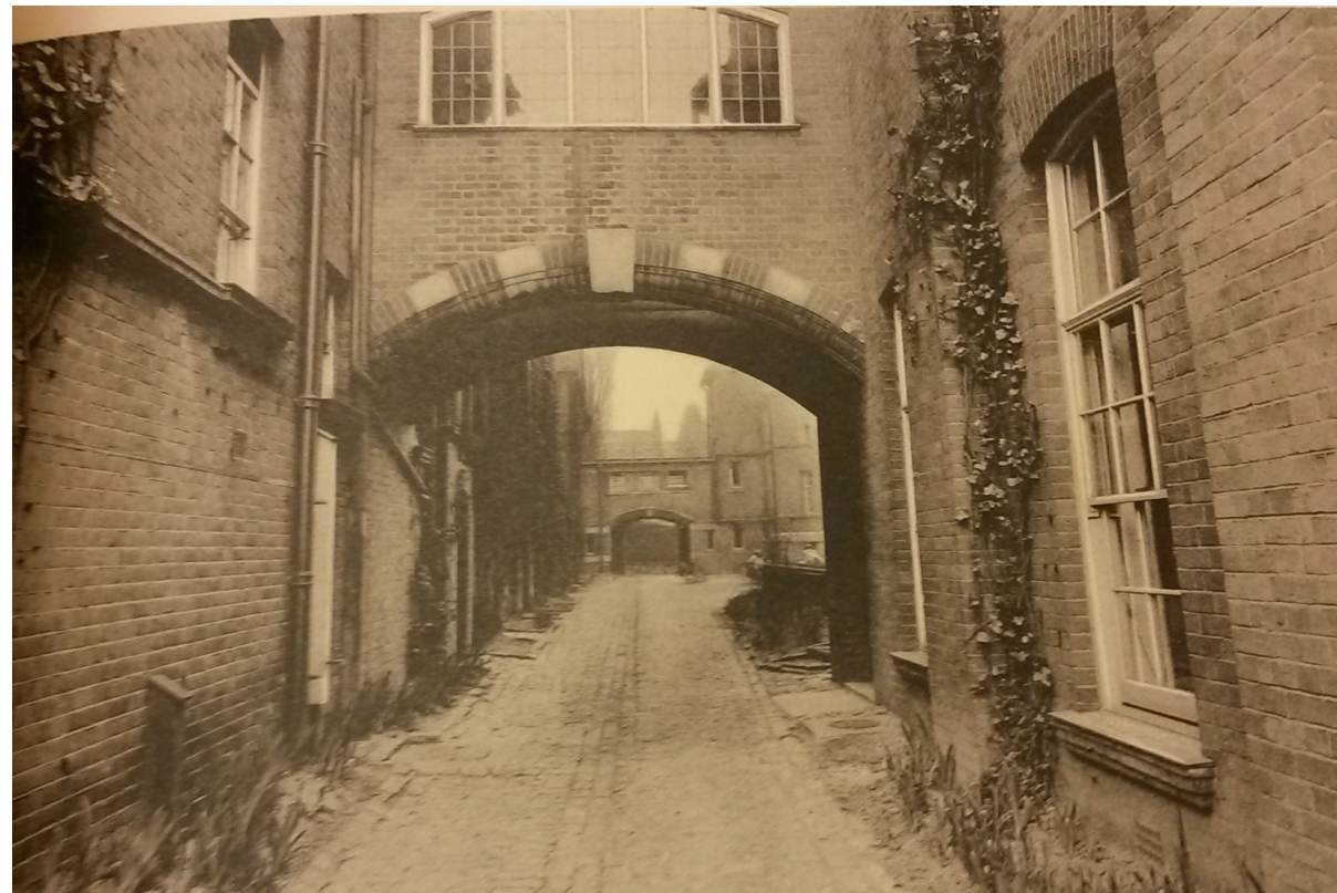
Figure 89. A photograph of the bridge structure which provided the original link between Skeel Library and Maynard Wing.
