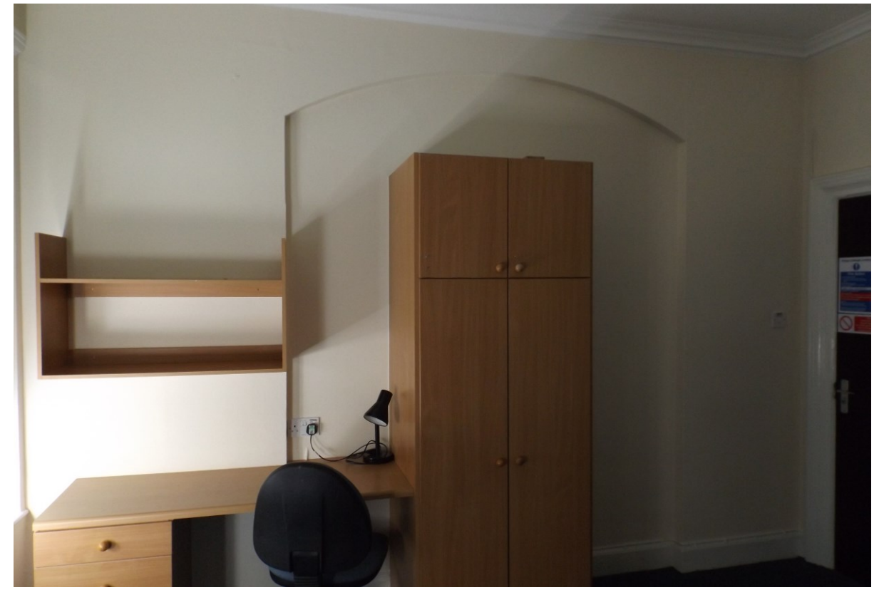
Figure 84 A typical student room. The infilled archway is an example of an original opening that has been infilled. The plans at Figure 78 provide evidence for this infill work carried out in 1973.
