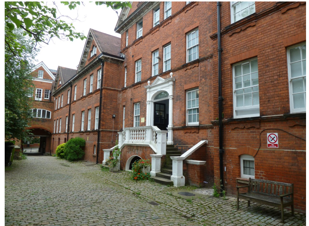
Figure 76 A photograph of the east elevation to the Maynard Wing photographed looking south with one's back to Lady Chapman Hall.
