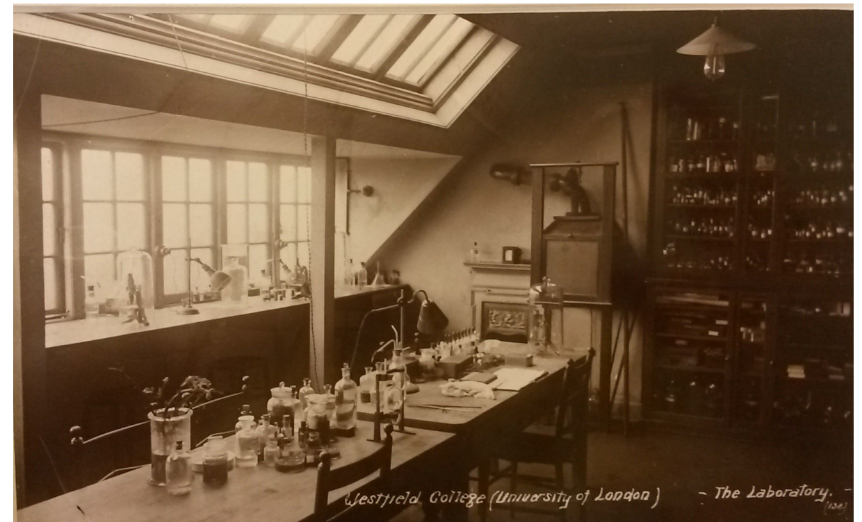
Figure 74 A photograph of the interior of the former laboratory building at the top of the Maynard Wing. This photograph appears to have been taken not long after the construction of the Maynard Wing.
