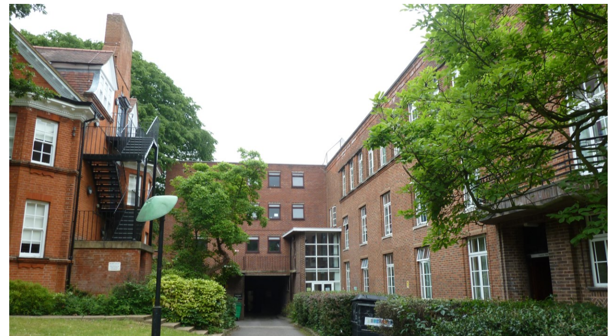
Figure 45 A view into the site from Kidderpore Avenue, showing the vehicular access into the basement parking level beneath Rosalind Franklin Hall.
