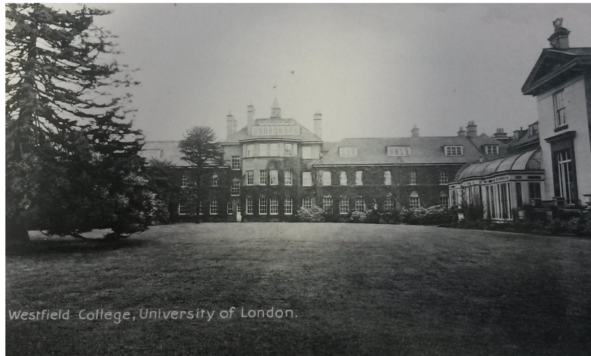
Figure 50 An image on a postcard c. 1905 of the lawn outside Kidderpore Hall prior to the demolition of the conservatory and its replacement with the 'Bay'.
