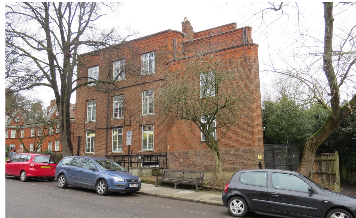
Figure 44 An image of Lord Cameron Hall looking into the site from a location almost opposite Lord Cameron Hall.
