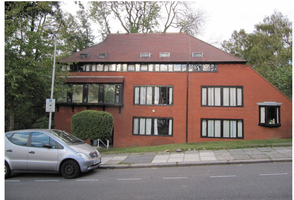
Figure 46 An image of Queen Mother's Hall as seen from Kidderpore Avenue, current date.
