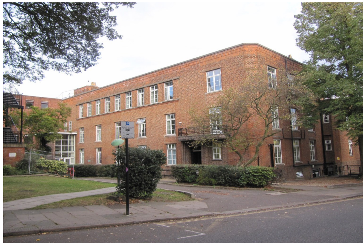
Figure 40 A photograph of the west and south elevations to Kidderpore Avenue
