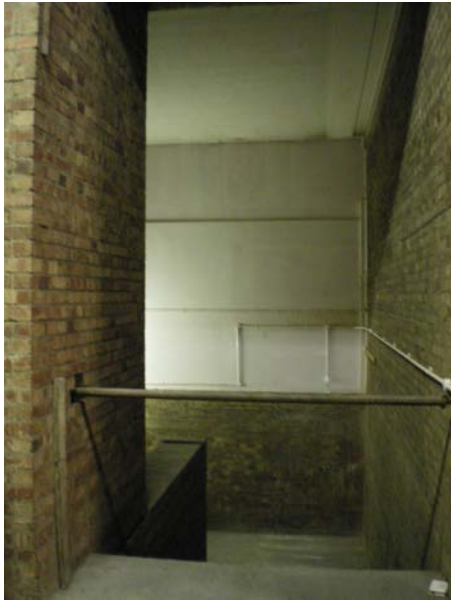
Figure 3 Location for new escape door in plaster-board partition
