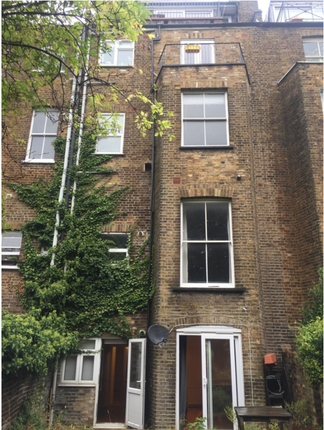
Photograph 1 – View of existing rear elevation
