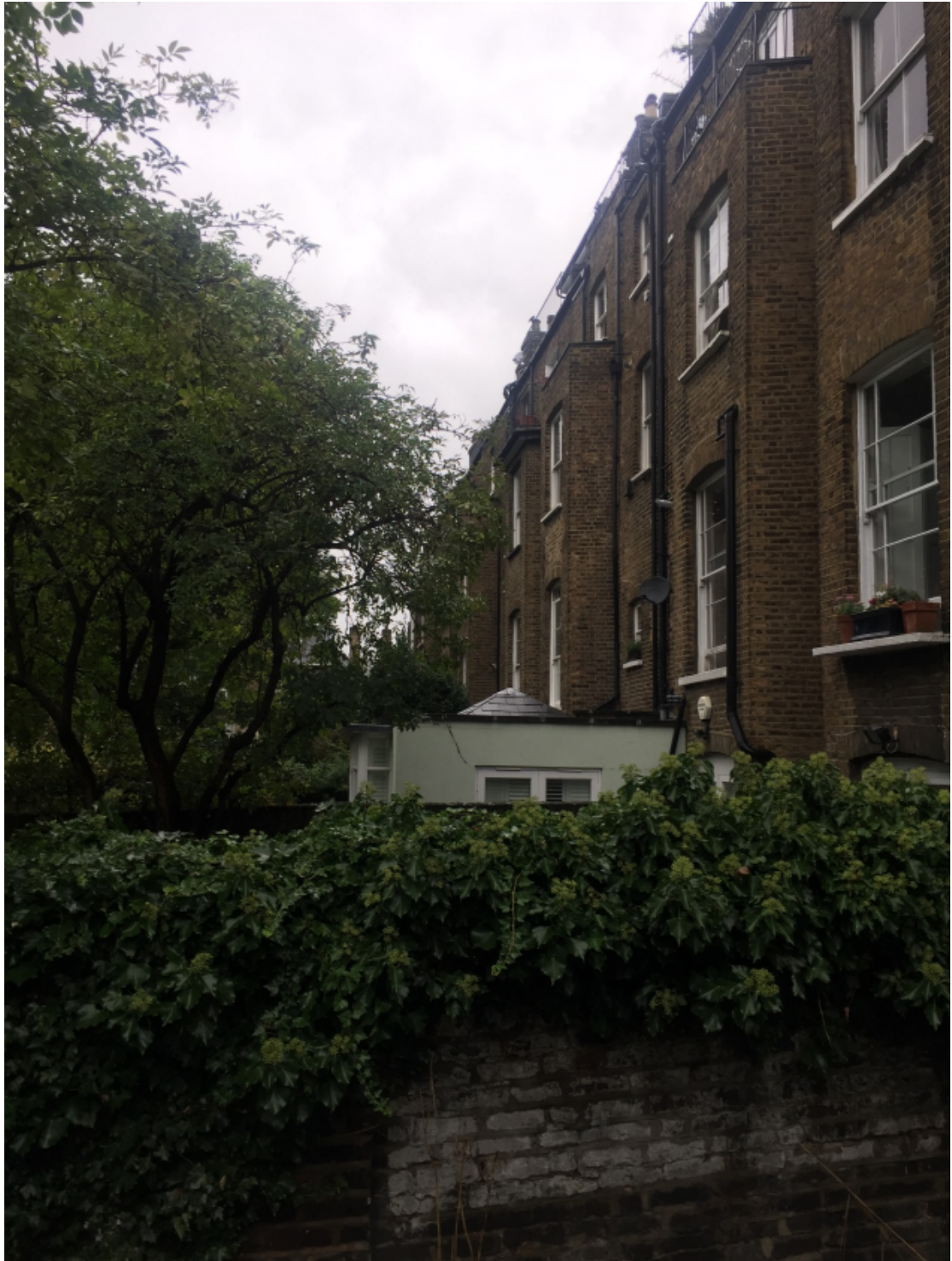
Photograph 2 – View of existing western neighbouring boundary.
