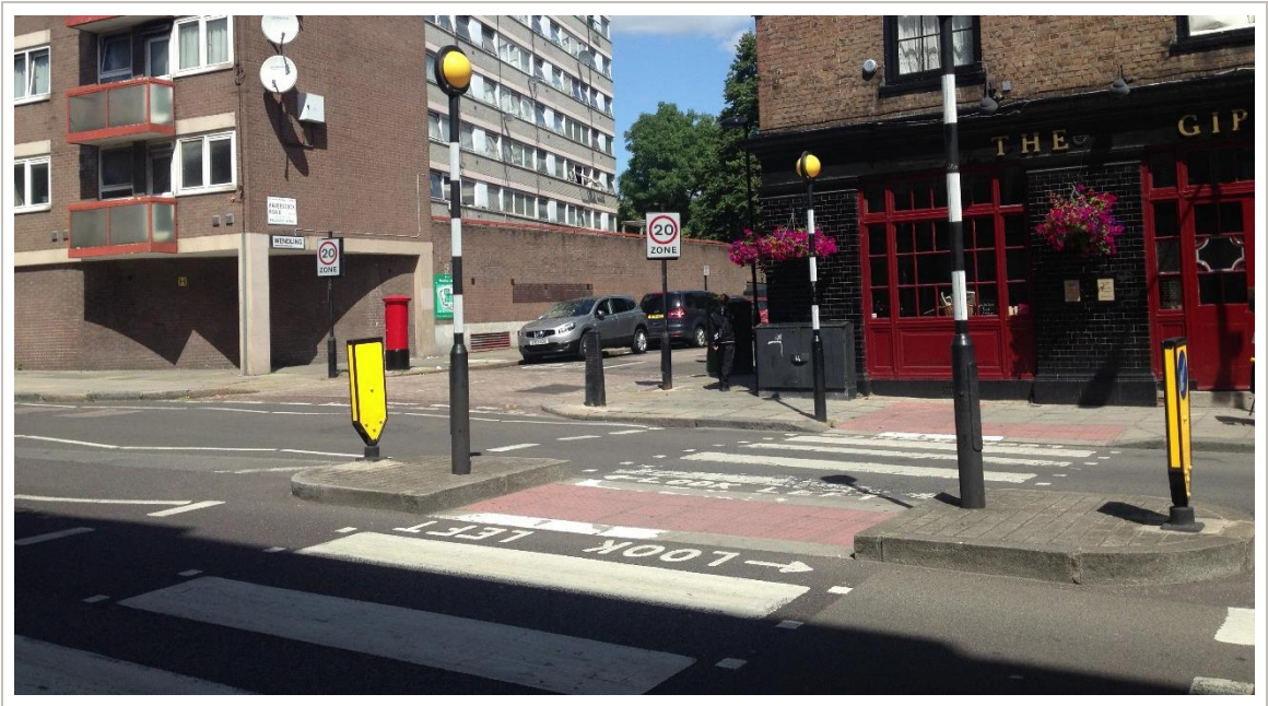
Figure 2.4 Pedestrian Crossing, Malden Road
