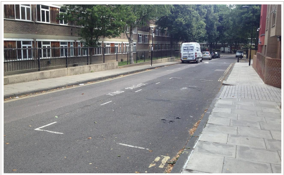
Figure 2.2 Wellesley Road Loading Bay
