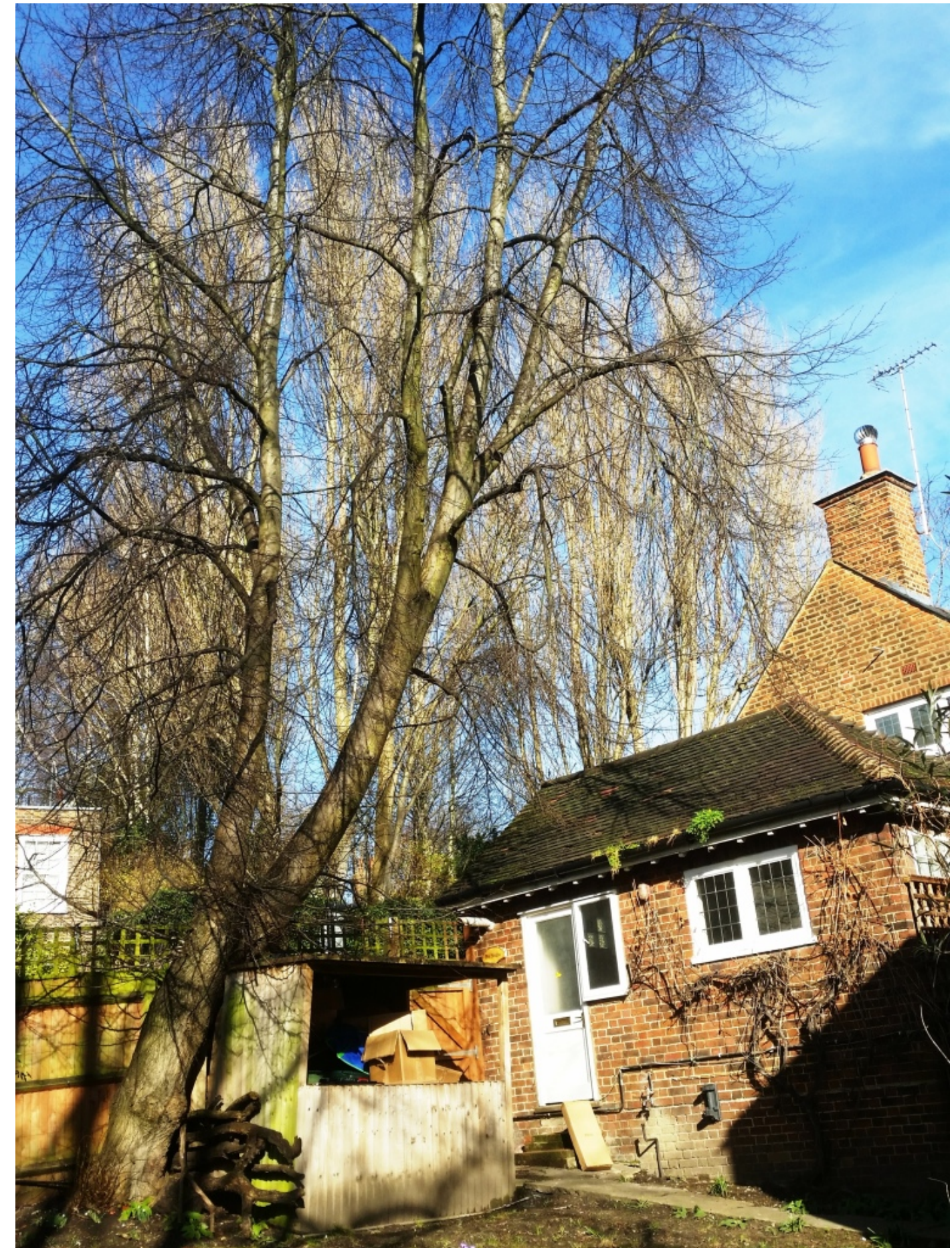
Lime T2 from existing patio next to house and showing lean towards the existing office building (proposed to become a garage)
