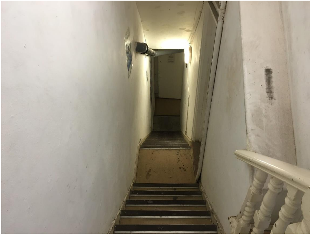
Photo 5: View of existing stair at No.61 TCR
