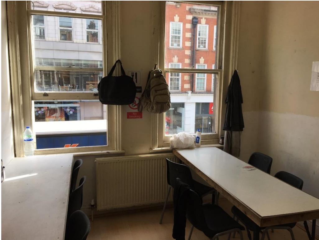
Photo 7: View of part of the site office at 1 st – 3 rd Floors at No.61 TCR
