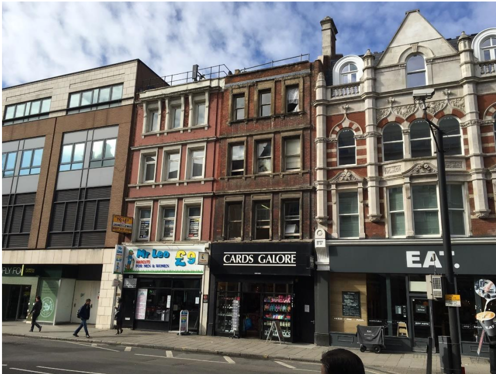
Photo 1: View of façade of Nos. 60 & 61 Tottenham Court Road
