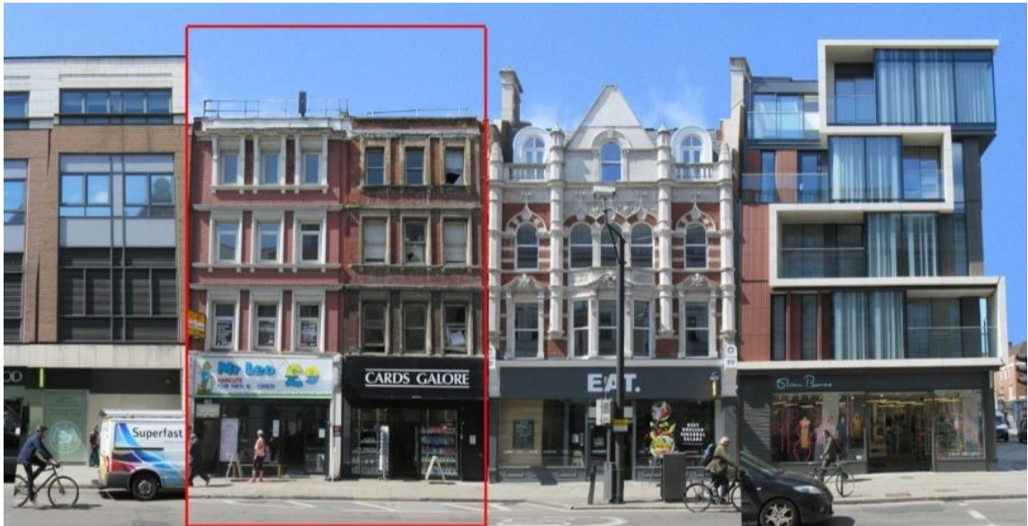
Figure 1.2: Existing buildings in street context
