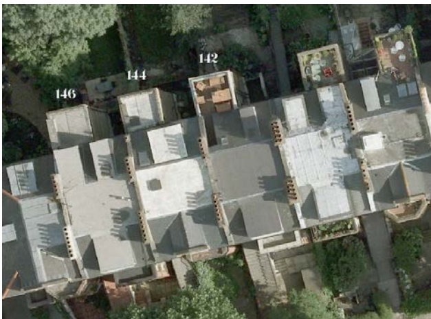
Aerial View showing neighbouring properties with varying means of access to the Annex roof, including a roof cut-in which at number 142
