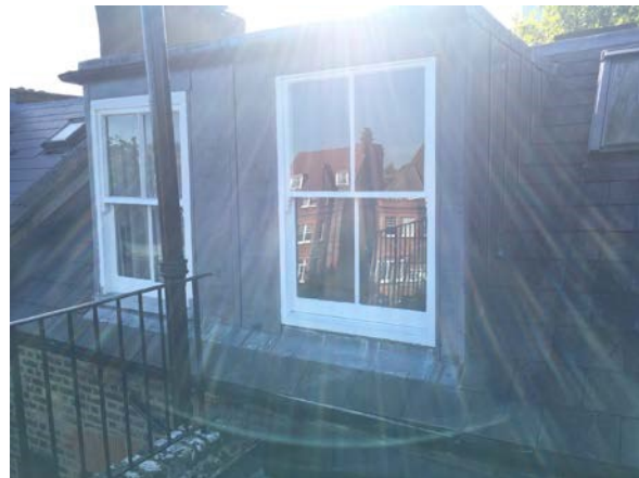
View of Existing Dormer at Rear of Building
