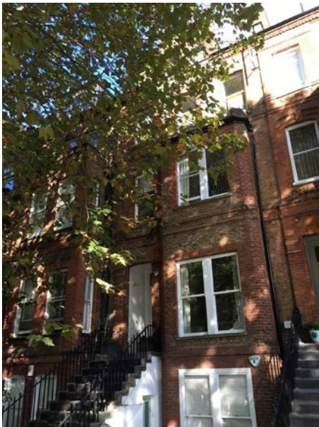
View of Front of Building from Fellows Road
