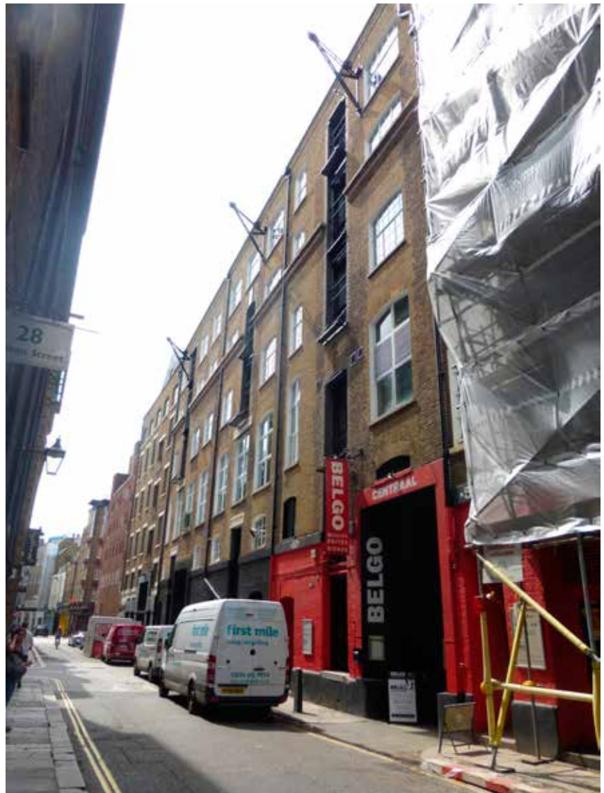
18. Side elevation of the Seven Dials Warehouse facing onto Shelton Street, 2016 (DIA)
