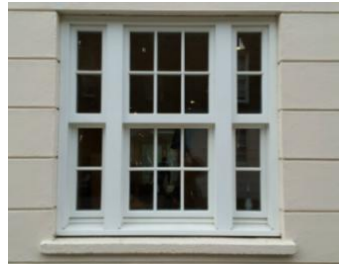
An example triple glazed sash window, in this case a casement lookalike, viewed from outside. © Passisash
