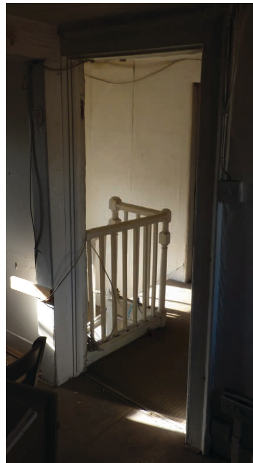
5 Photo of Existing Door Frame 3F N.T.S.
