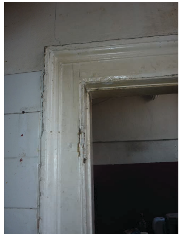
5 Photo of Existing Door Frame 1F N.T.S.
