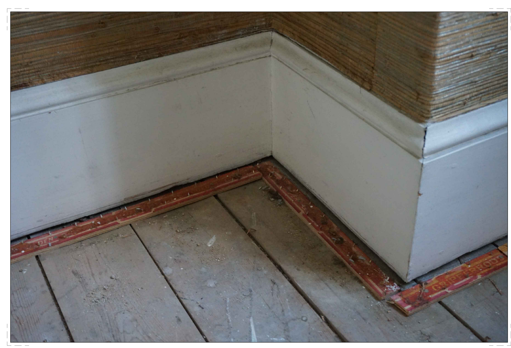
Typical Existing Skirting to be Replaced
