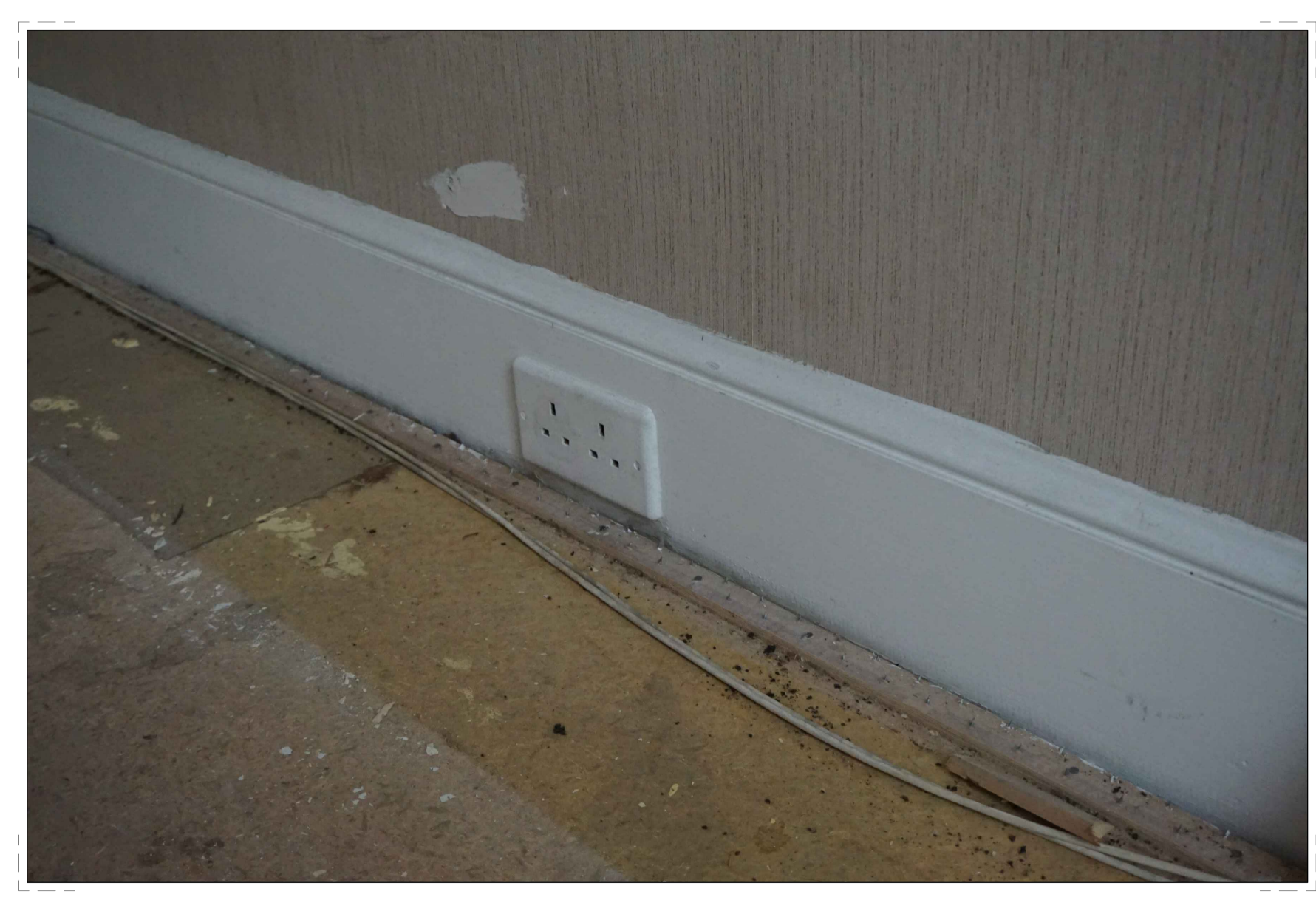
Typical Existing Skirting to be Replaced
