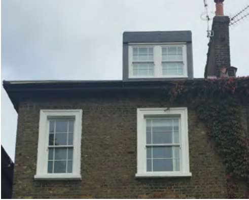
Image 1.02- 22 Rochester Square- Existing front elevation of the house with a double lead clad dormer
