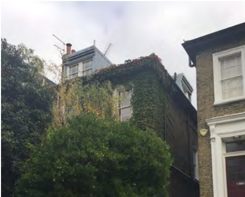
Image 1.03- 21 Rochester Square- Existing front and side double lead clad dormer
