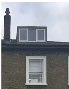
Image 1.07(left)- 16 Rochester Square- Existing front double lead clad dormer
