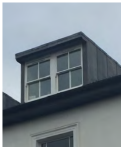
Image 1.05(left)- 18 Rochester Square- Existing front double lead clad dormer
