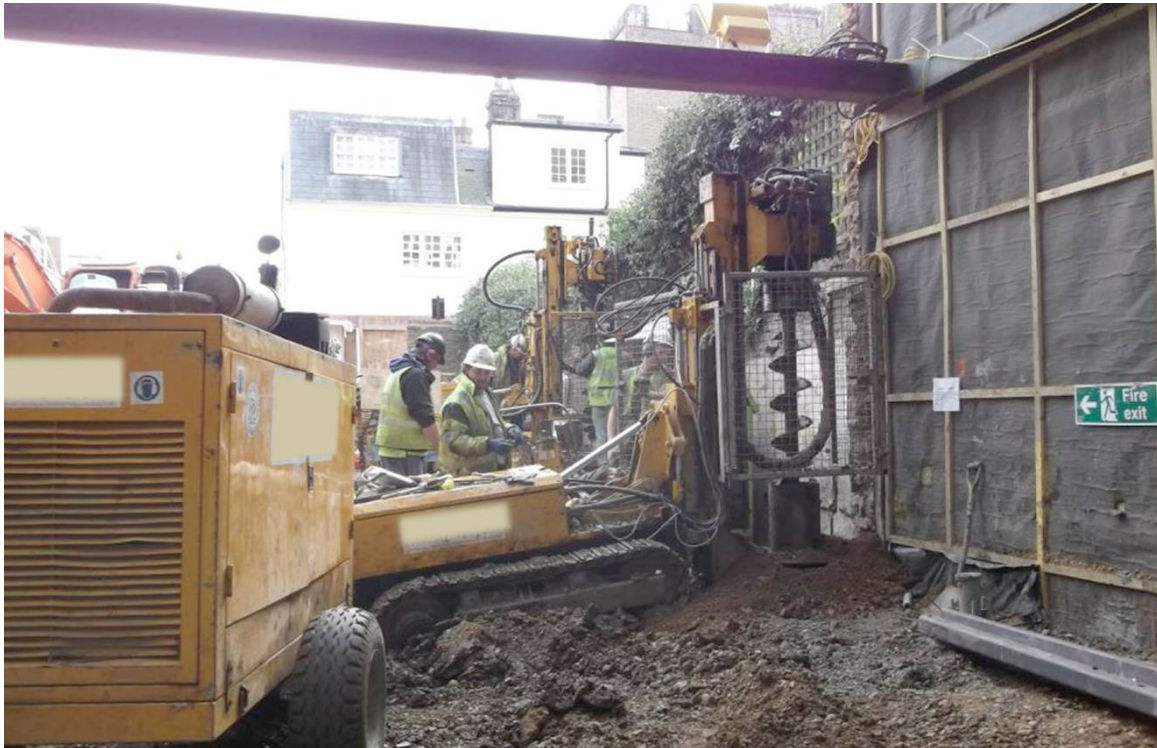
Figure 4 Piling rig at work within basement
