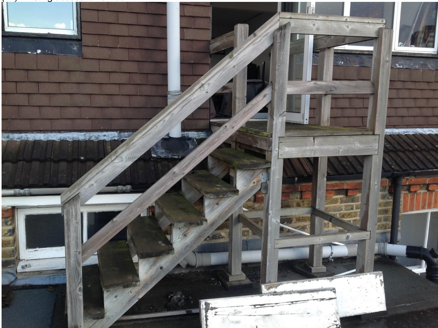
(11) Existing access to flat roof.
