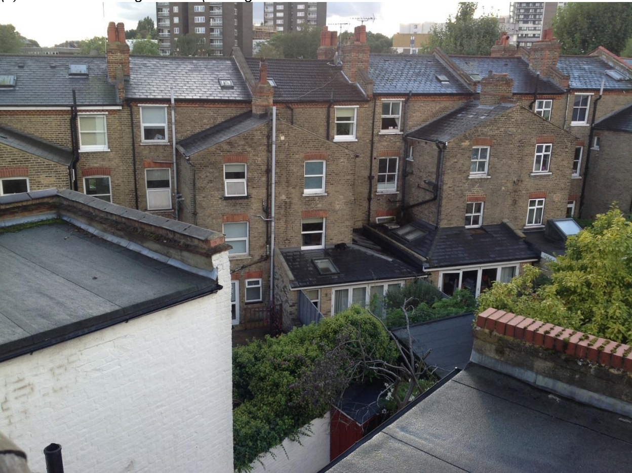
(8) View from existing flat roof (looking South)
