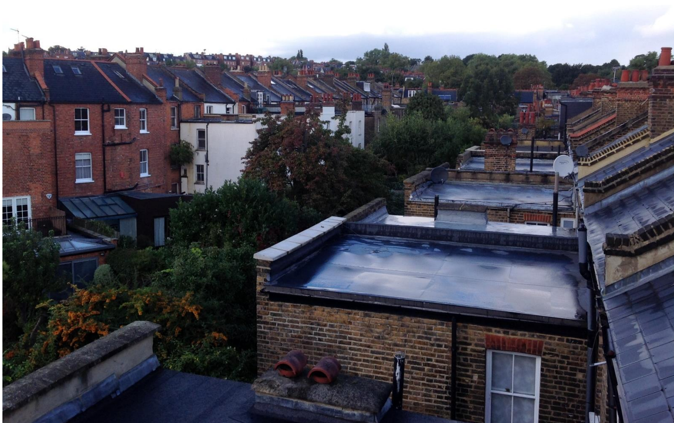
(6) View from existing flat roof (looking North)
